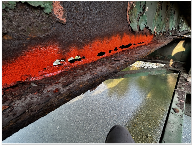
Downstream fascia stringer node 3 end
