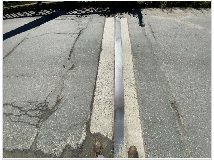
Abutment 2 joint
