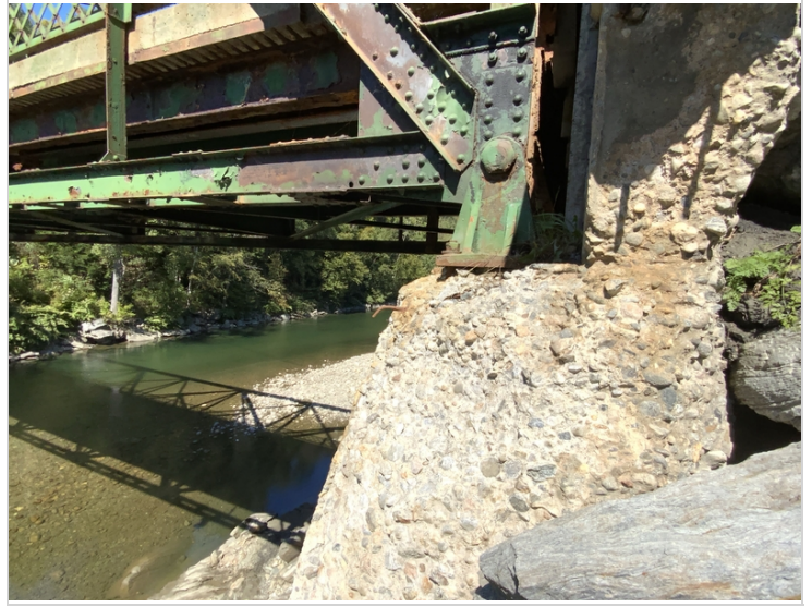
Abutment 1 upstream bearing
