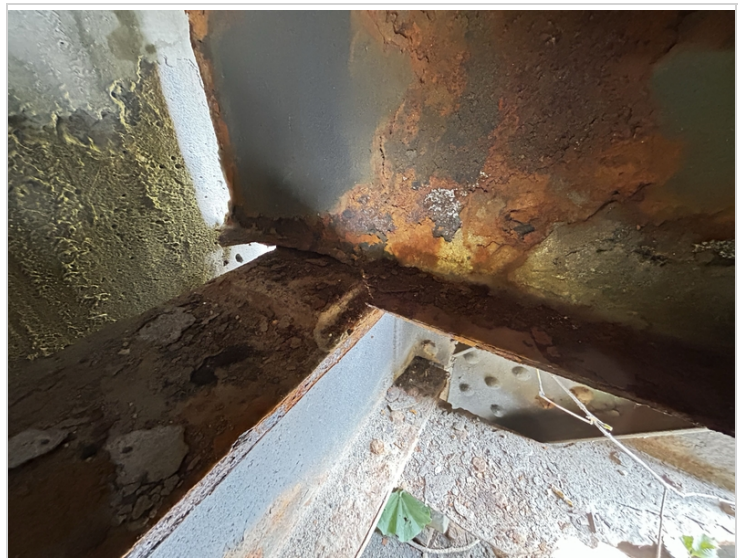
Stringer 5 (downstream fascia) abutment 2
