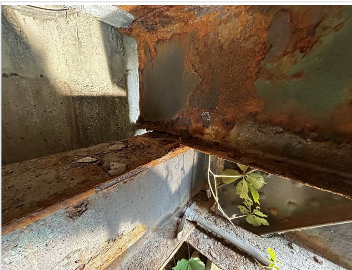
Stringer 5 (downstream fascia) abutment 2
