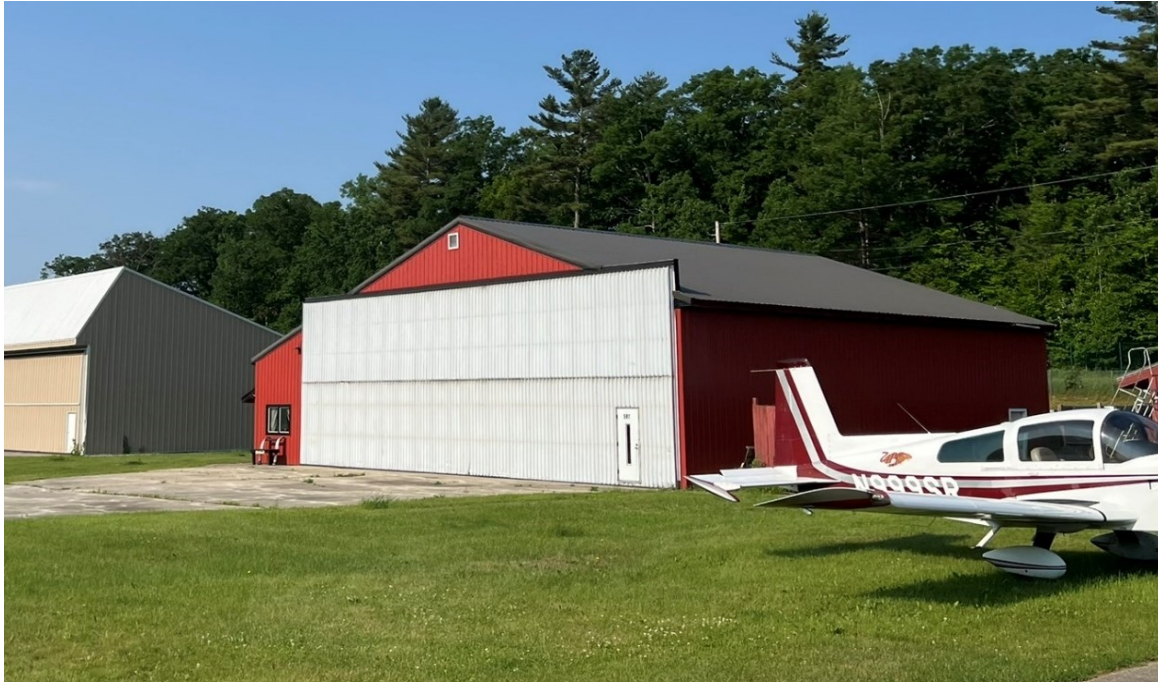
Photo 20. View of Resource 16 looking southwest.
