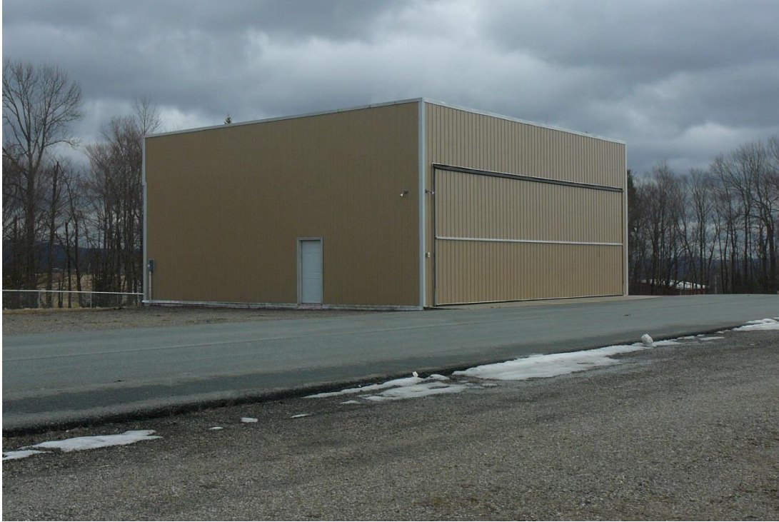
Figure 16. View southeast of the southernmost hangar at the Caledonia County State Airport.
