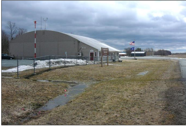
Caledonia County State Airport Terminal
