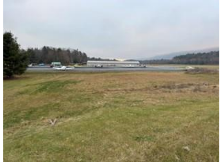
North Terminal – looking north across project area
