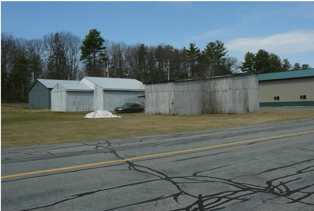
Figure 83. View northwest of hangars at the Middlebury State Airport; T-hangars at right and center.
