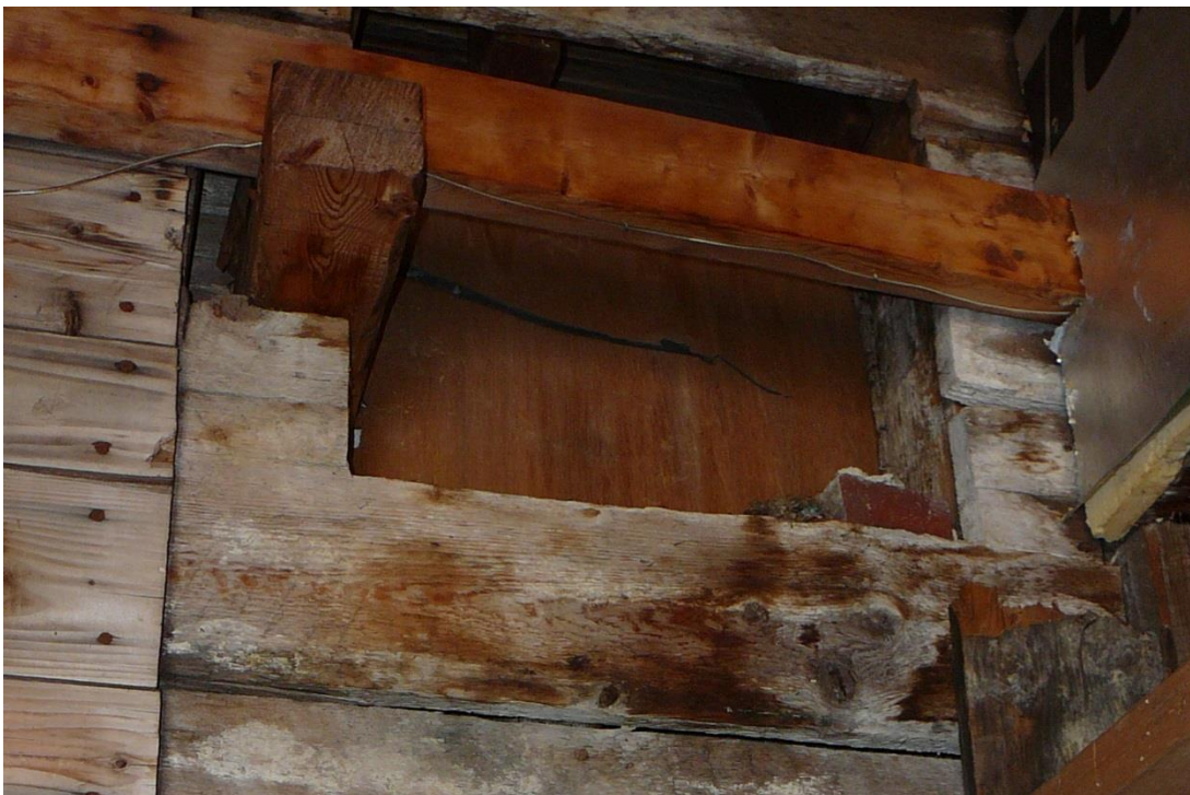
Figure 42. Exposed wood sheathing along the west wall of the main block of the Pudding Hill School, visible from within the addition; the wall may be a former exterior wall with a window opening, in place prior to the construction of the addition.
