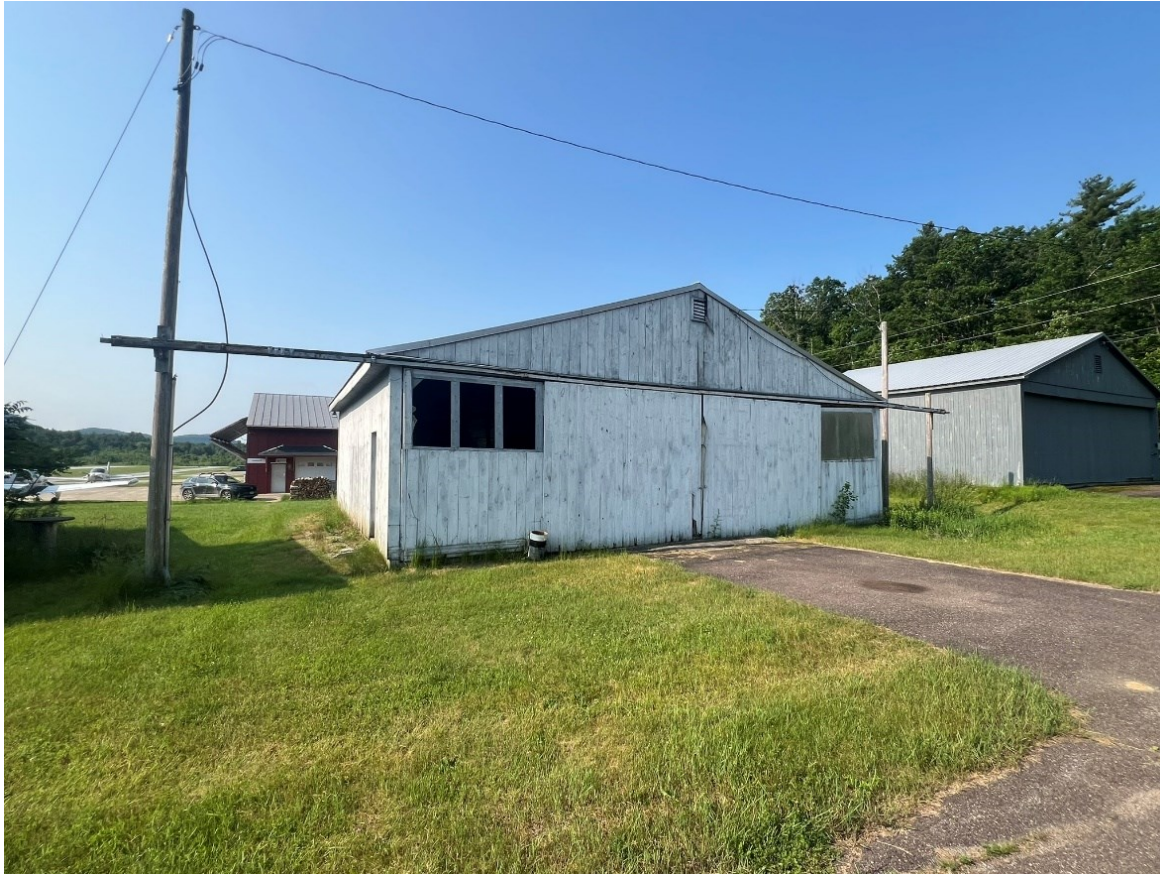
Photo 17. View of Resource 13 looking southwest.
