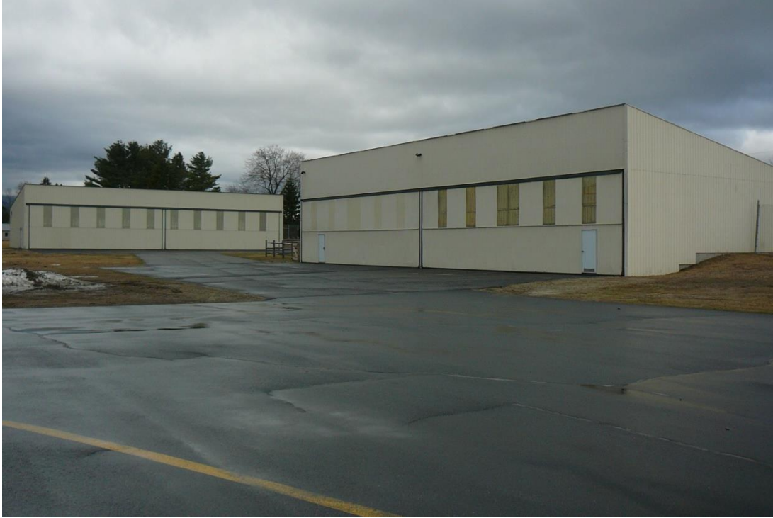
Figure 104. View southwest of hangars at the southern end of the Morrisville-Stowe State Airport.
