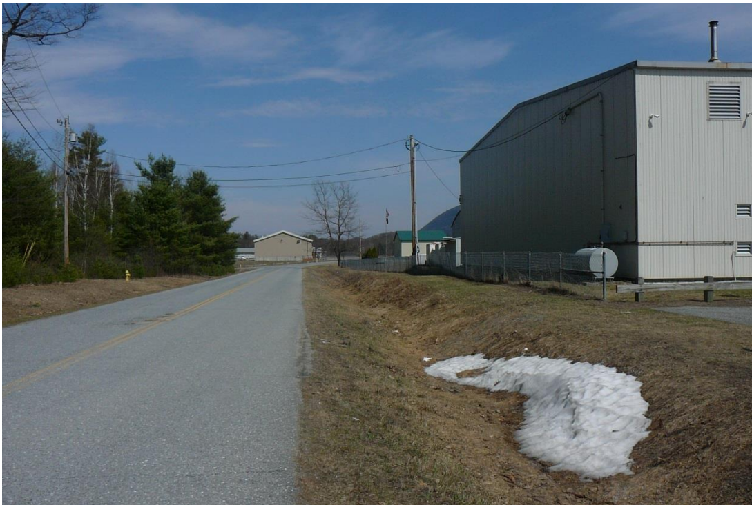
Figure 63. View north of Middlebury State airport along Airport Road.
