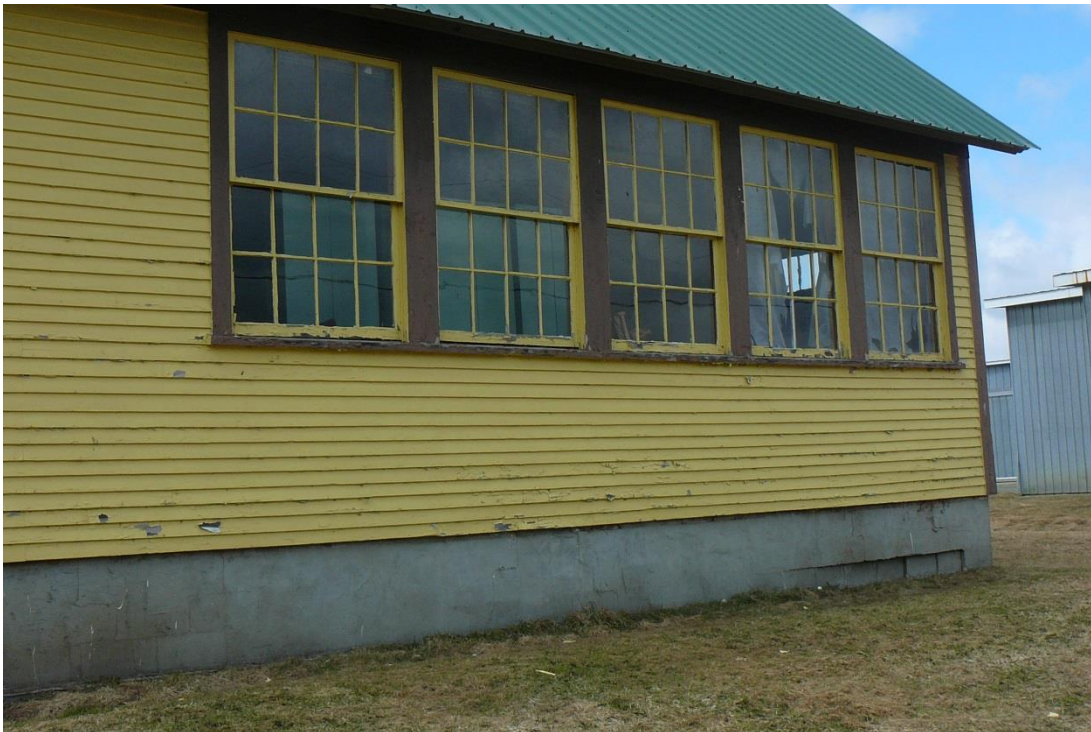
Figure 31. View of windows along the east elevation of the Pudding Hill School at the Caledonia County State Airport.
