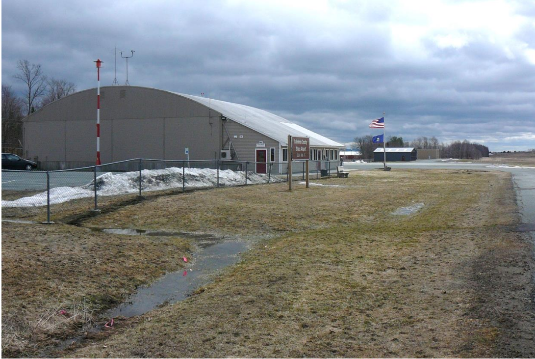
Figure 10. View southeast of buildings at the Caledonia County State Airport.
