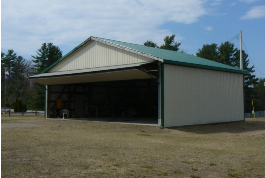
Figure 76. View southwest of hangar at the Middlebury State Airport.
