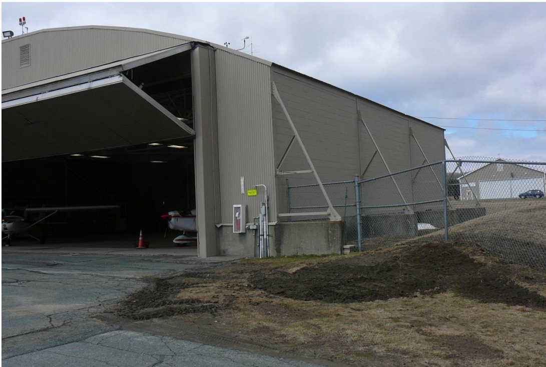
Figure 47. View northwest of terminal/Esline hangar at the Caledonia County State Airport.
