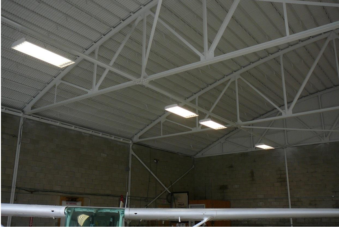
Figure 50. View of interior metal frame in terminal/Esline hangar at the Caledonia County State Airport.
