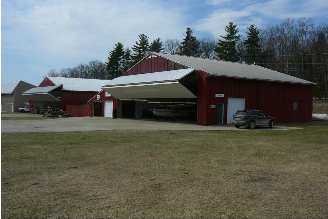
Figure 84. View southwest of hangars at the Middlebury State Airport
