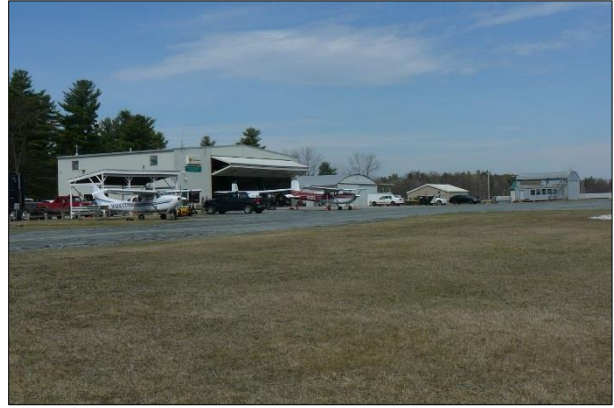
Middlebury State Airport Terminal
