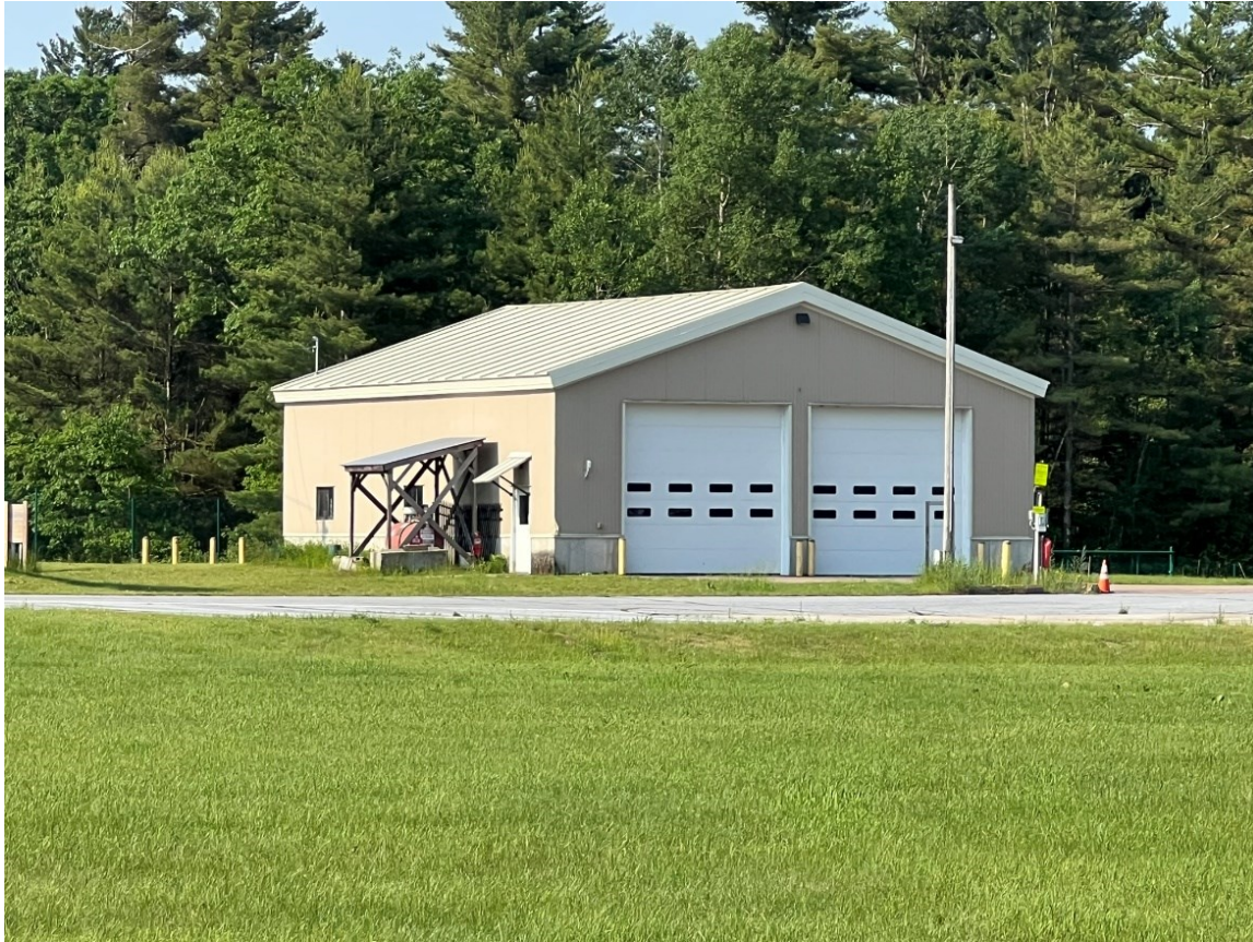
Photo 6. View of Resource 2 looking southwest.
