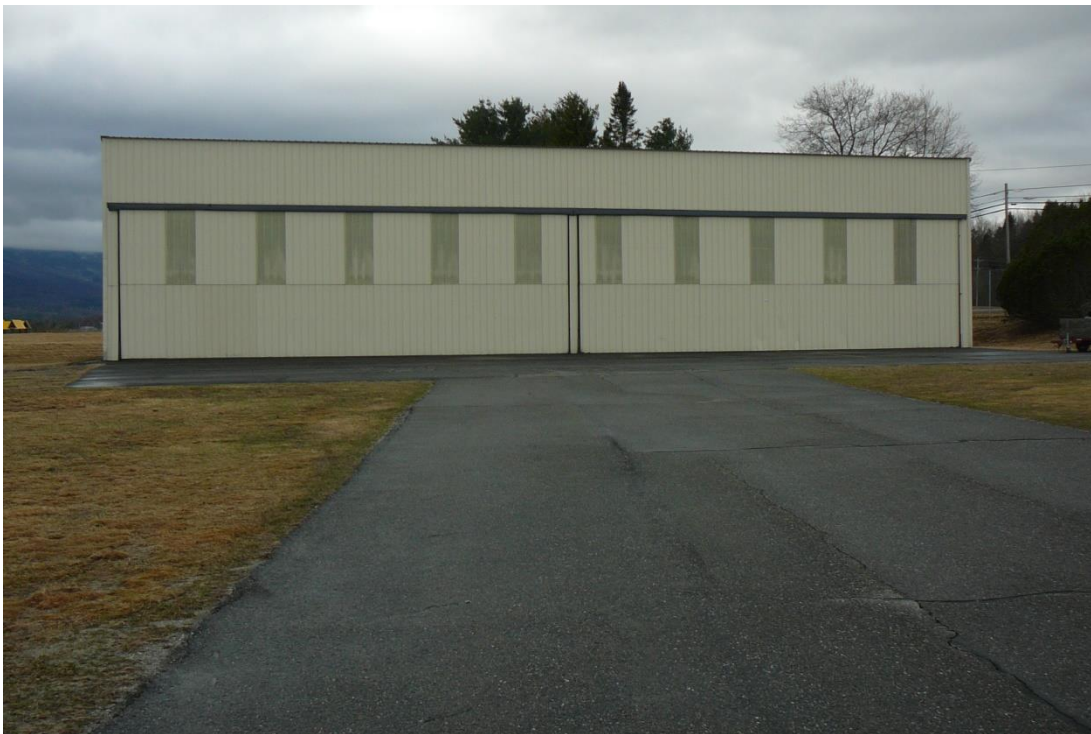
Figure 105. View southwest of southernmost hangar at the Morrisville-Stowe State Airport.
