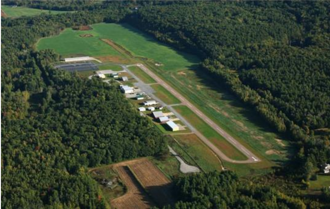
Figure 62. Aerial view of the Middlebury State airport, facing northeast ( http://vtrans.vermont.gov/aviation/airports/middlebury )
