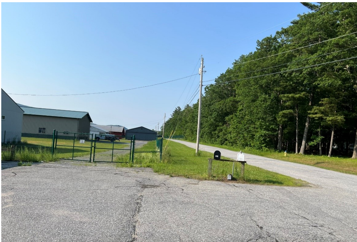
Photo 2. View of Airport Road looking south.
