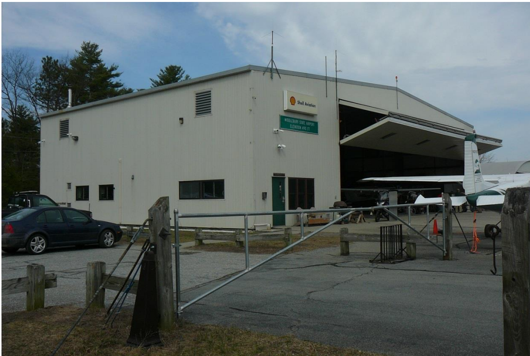
Figure 79. View northwest of terminal/hangar at the Middlebury State Airport.
