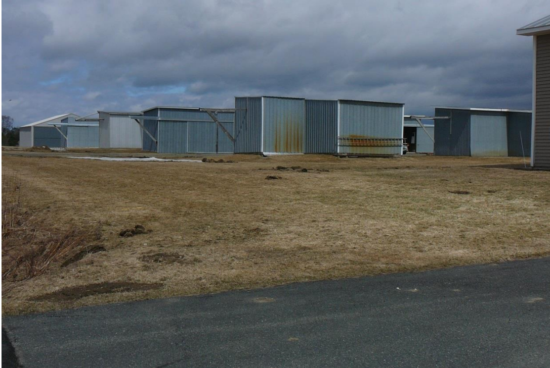
Figure 18. View northeast of T- hangers at the Caledonia County State Airport.
