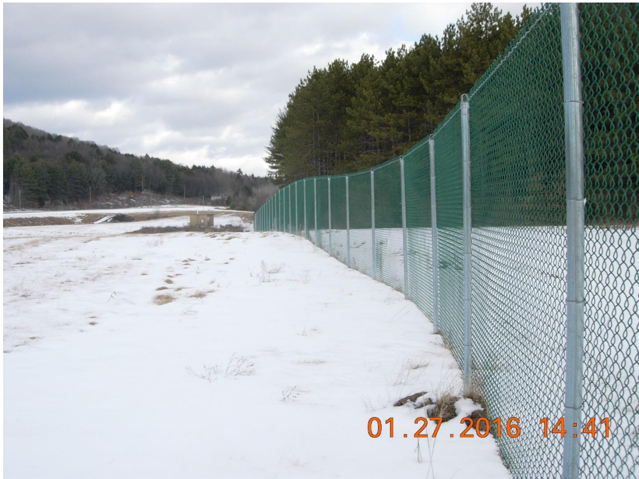
Figure 2. Image of typical chain link fencing to be installed during project work (image provided by VTrans).
