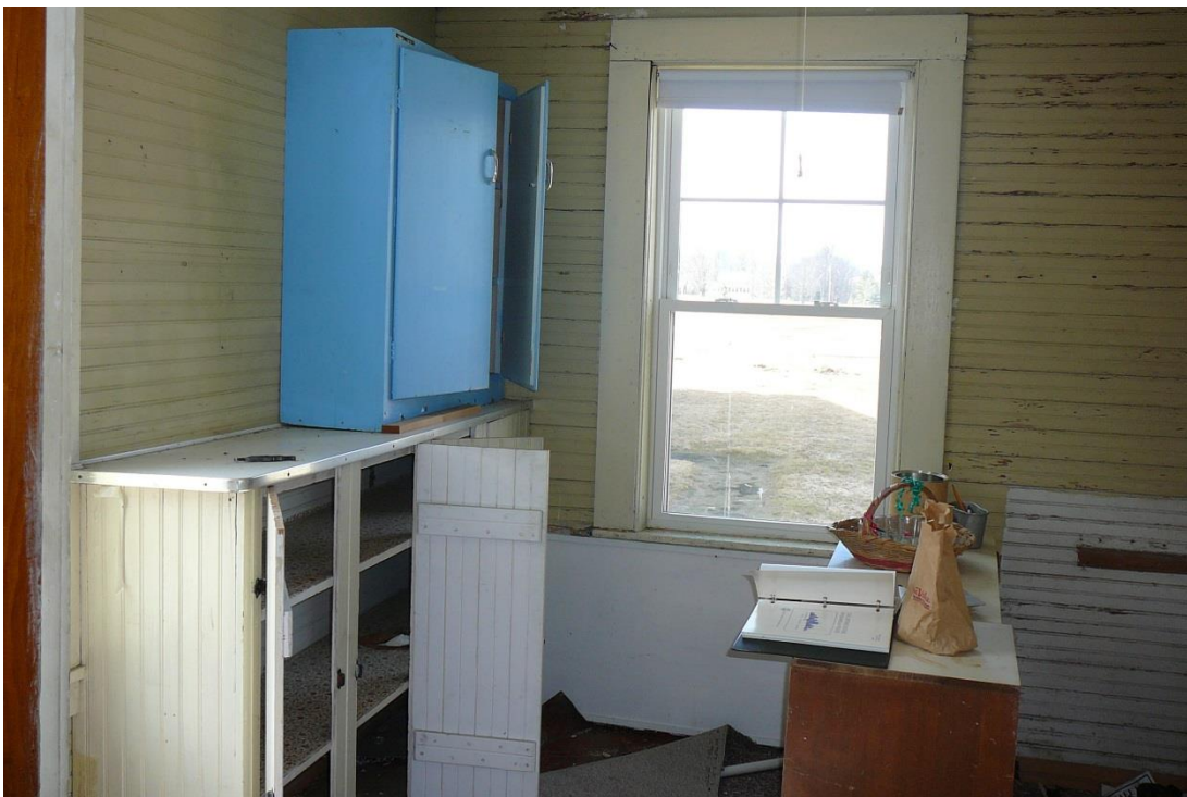
Figure 39. Small room in addition at the Pudding Hill School; note built-in cabinets and bead board wall covering.
