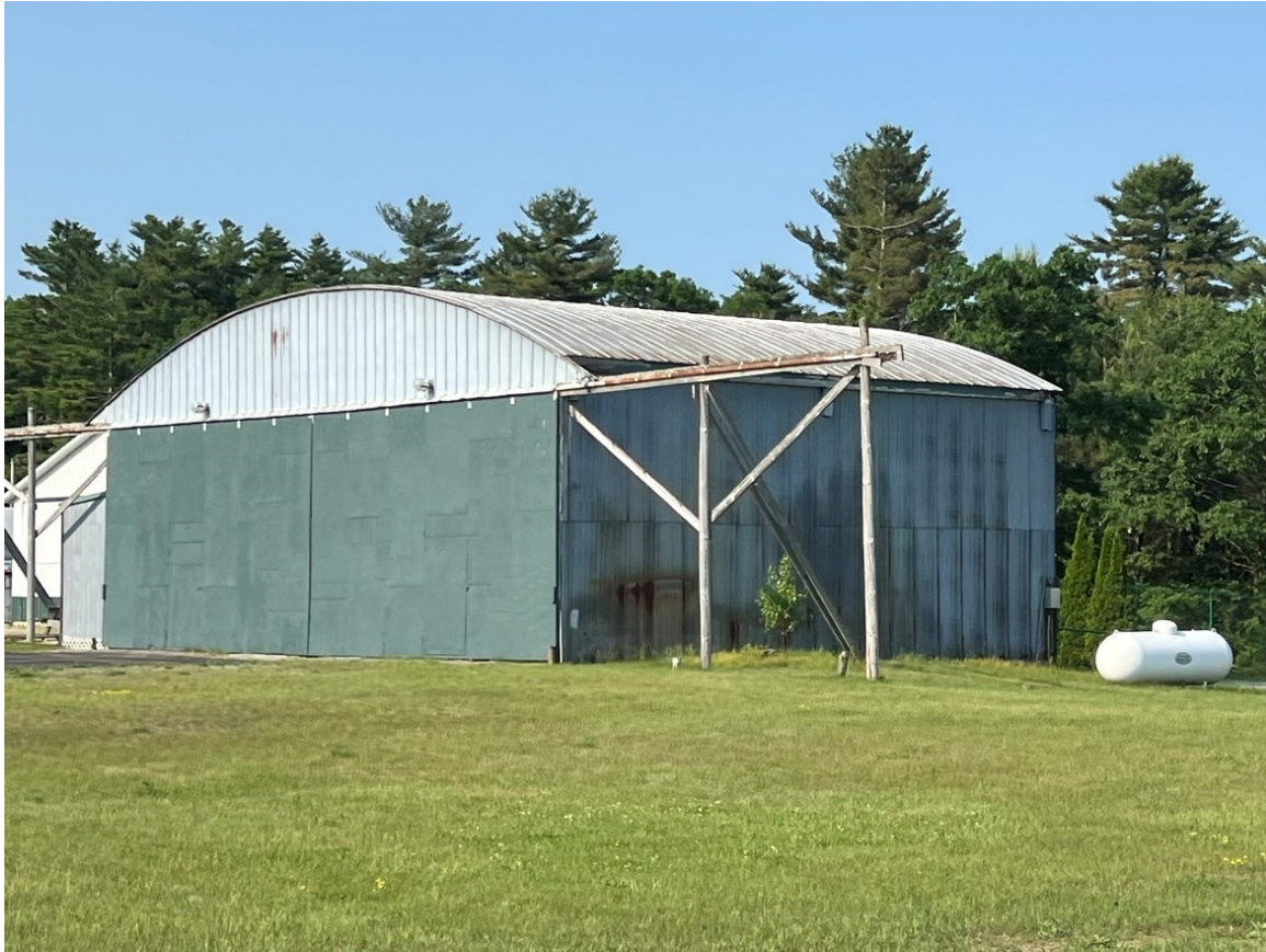
Photo 9. View of Resource 5 looking southwest.
