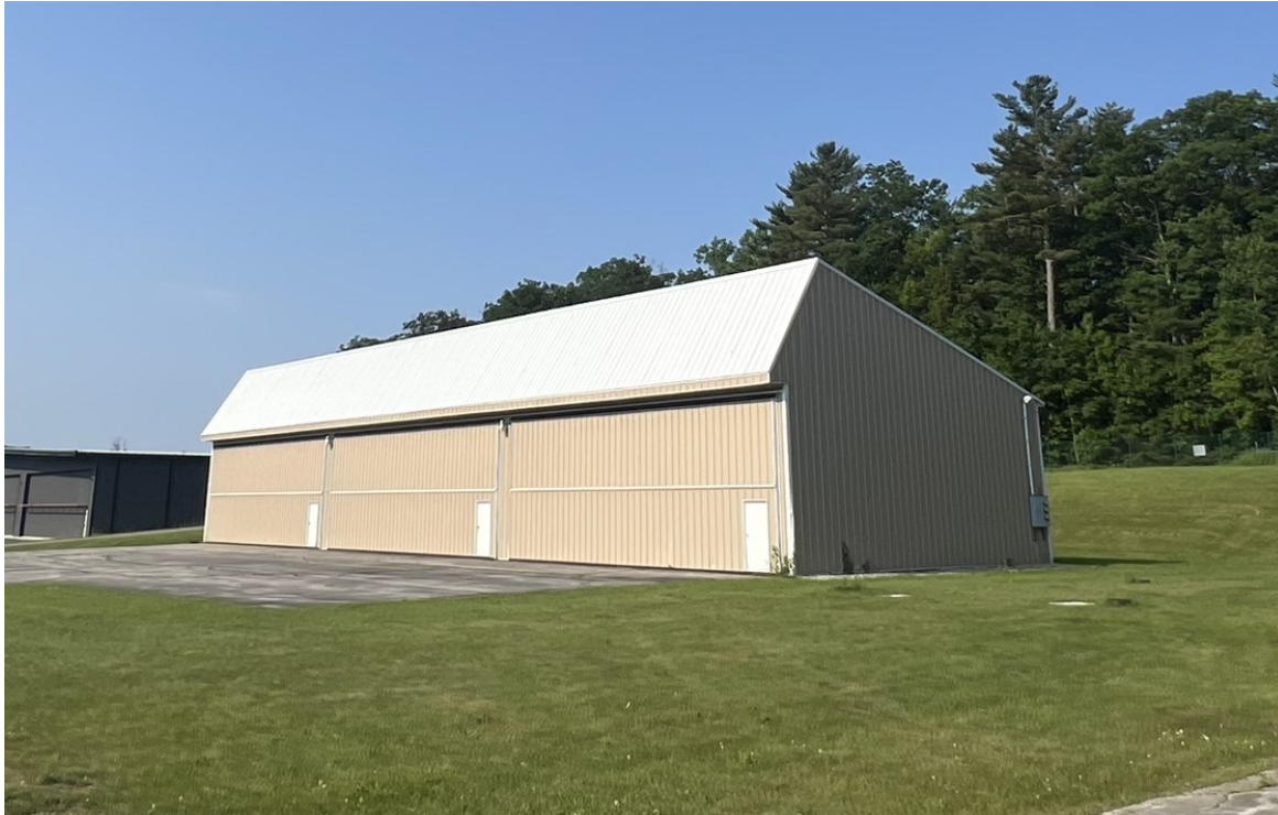
Photo 21. View of Resource 17 looking southwest.
