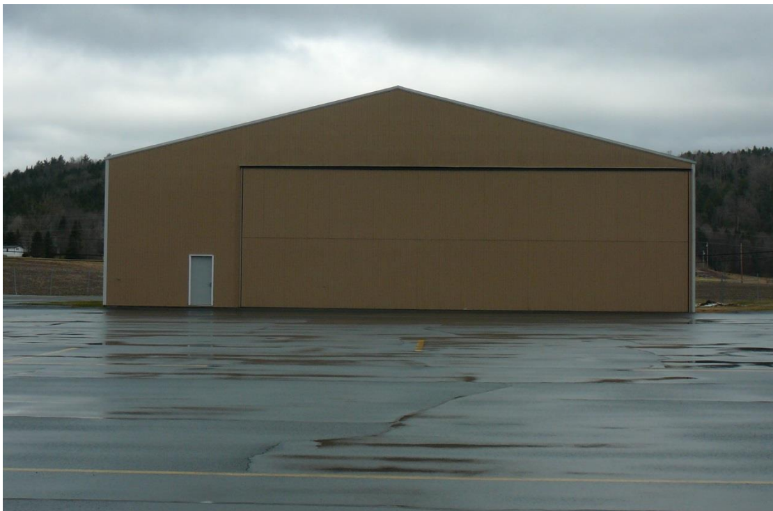
Figure 100. View west of hangar at the Morrisville-Stowe State Airport.
