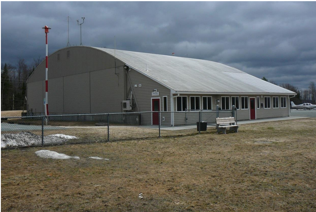
Figure 49. View southeast of terminal/Esline hangar at the Caledonia County State Airport.
