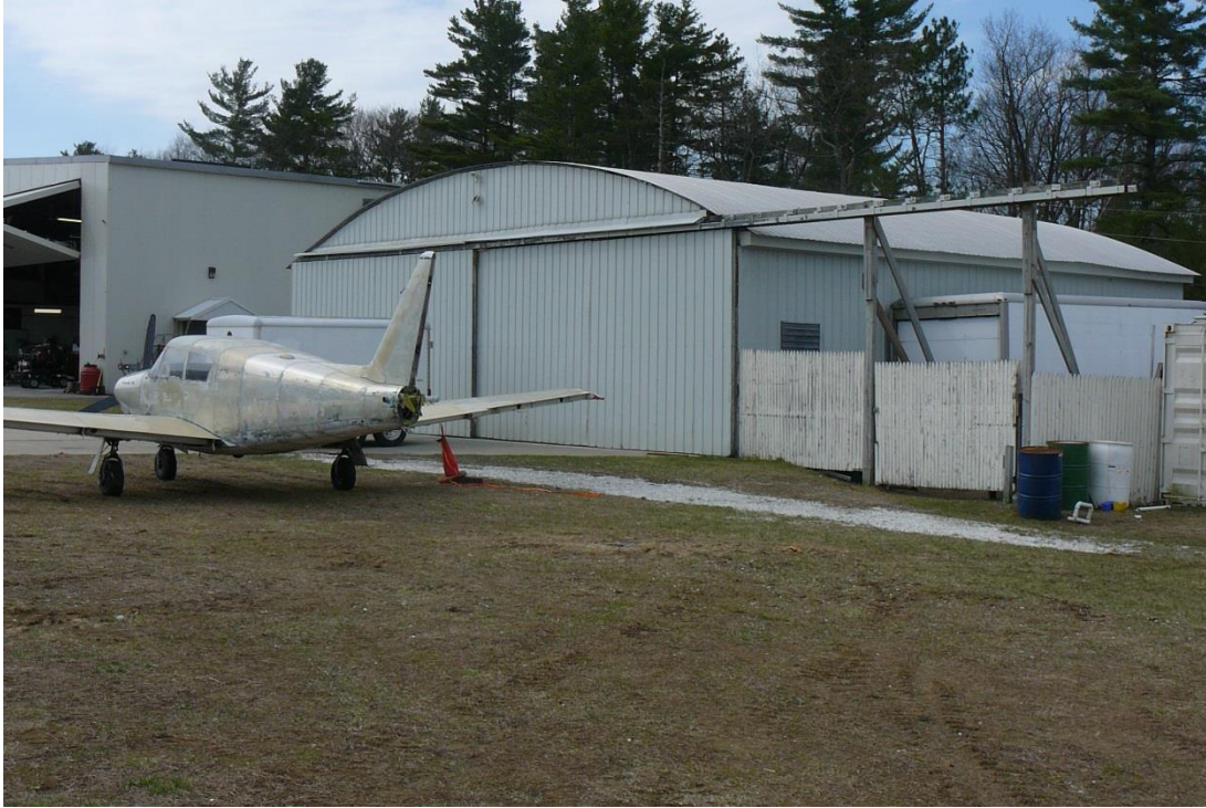
Figure 78. View southwest of smaller arched roof hangar at the Middlebury State Airport.
