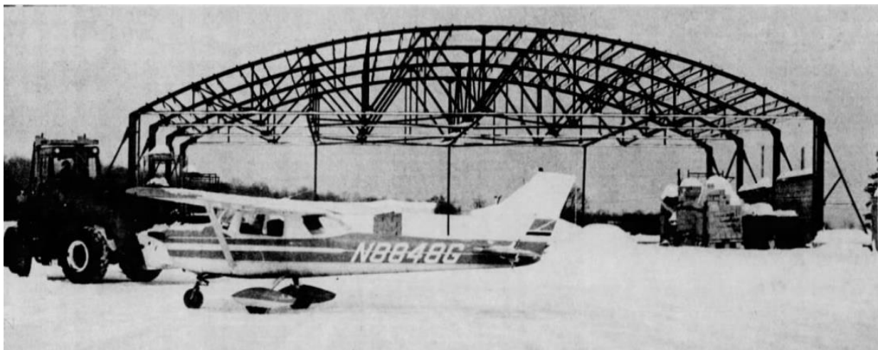
Figure 45. The old Burlington Esline hangar being rebuilt at the Caledonia County State Airport in Lyndon in 1976 ( Burlington Free Press February 15, 1976, photo credit Jan Herman).
