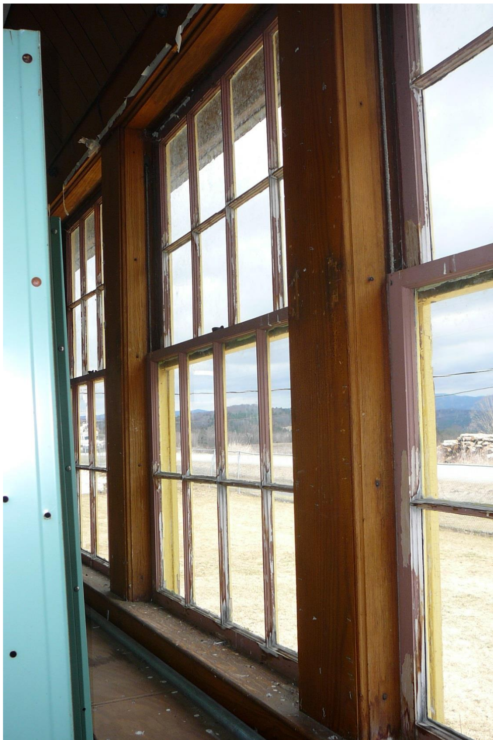
Figure 37. View north of bank of windows along east wall of the main room in the Pudding Hill School.
