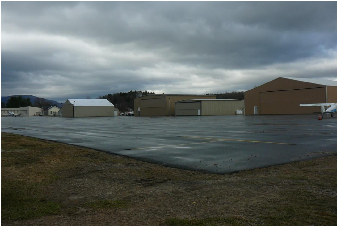
Figure 95. View southwest of buildings at the Morrisville-Stowe State Airport.
