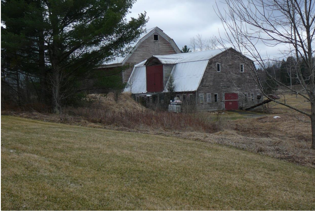
Figure 118. View southwest of gambrel roof barns at the former Malvern Farm location on the west side of VT Route 100.
