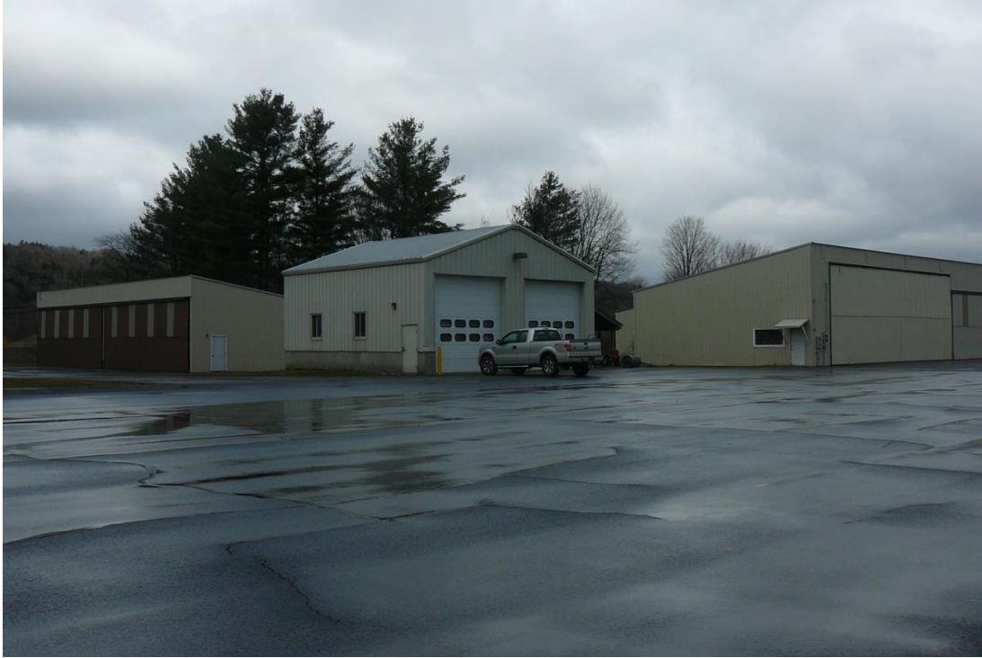
Figure 98. View northwest of hangars and garage at the northern end of the Morrisville-Stowe State Airport.
