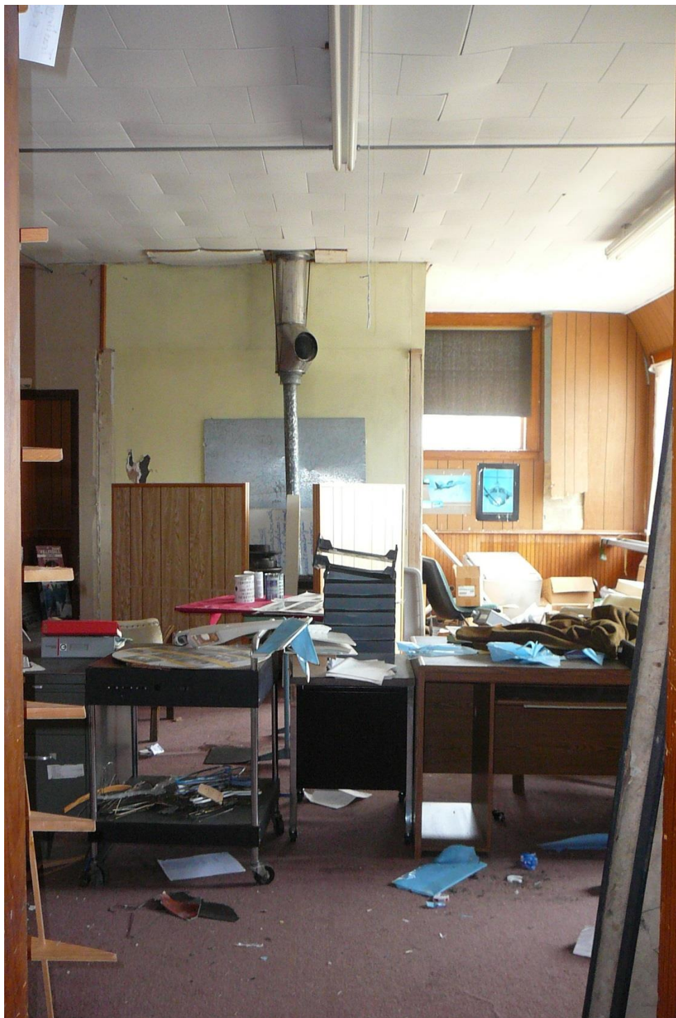
Figure 36. View toward the north wall of the main room in the Pudding Hill School, from the enclosed entryway.
