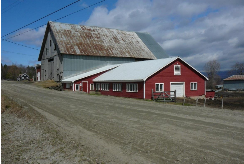
Figure 58. View northeast of the barn complex at the Proctor farm complex on the east side of Pudding Hill Road.
