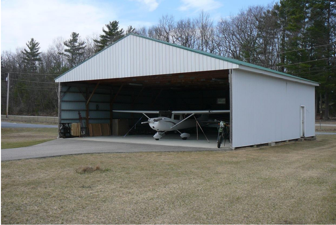
Figure 80. View southwest of hangar at the Middlebury State Airport.
