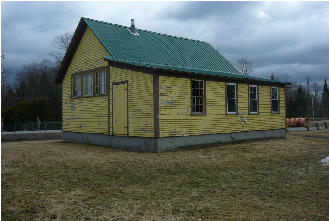
Figure 29. View southeast of the Pudding Hill School at the Caledonia County State Airport.
