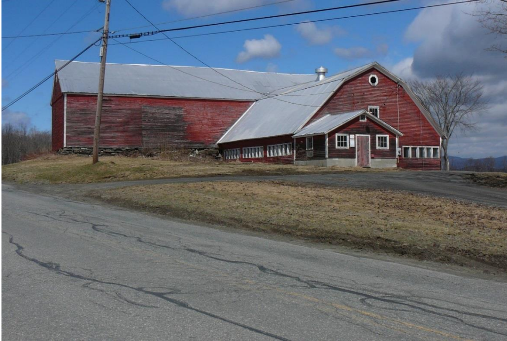
Figure 59. View northeast of the main barn complex at the Ruggles farm complex on the east side of Pudding Hill Road.
