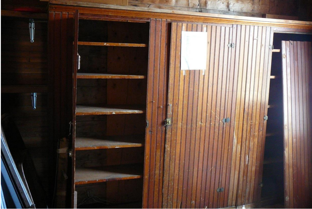
Figure 38. Built-in cabinets in small room in addition at the Pudding Hill School.
