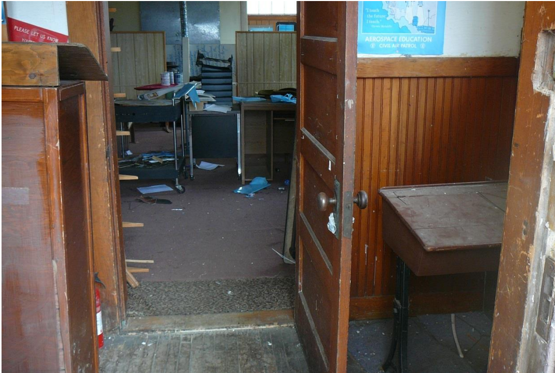
Figure 32. View north into the Pudding Hill School from the main entry door; entryway in foreground.
