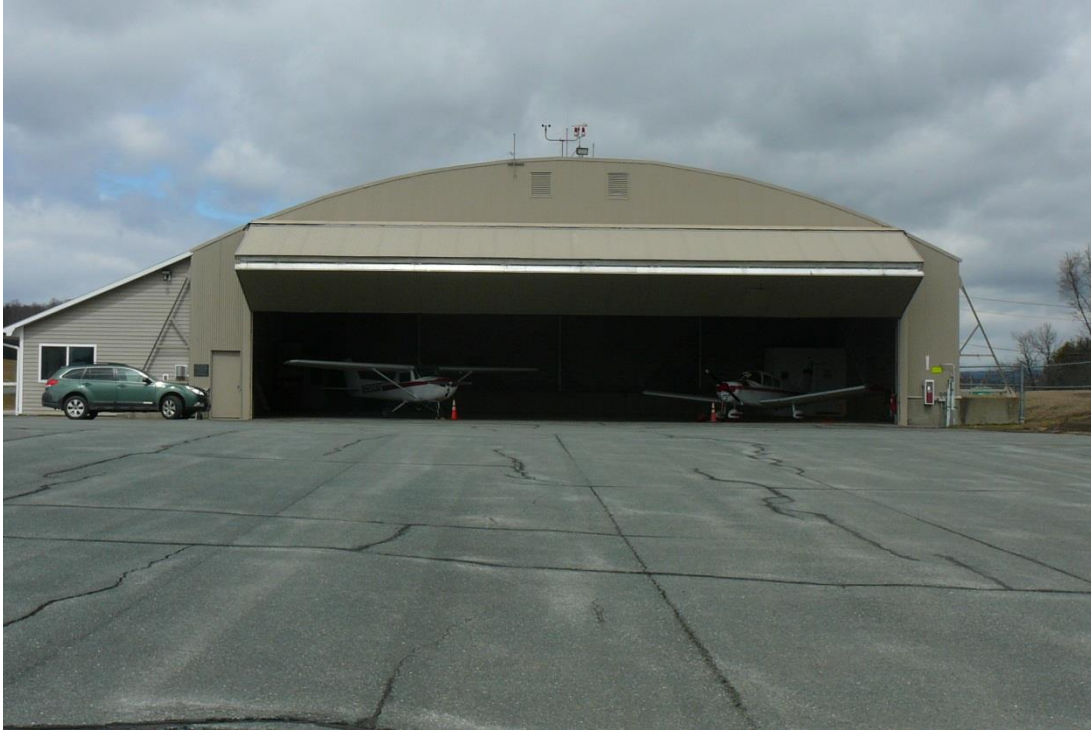
Figure 46. View north of terminal/Esline hangar at the Caledonia County State Airport.
