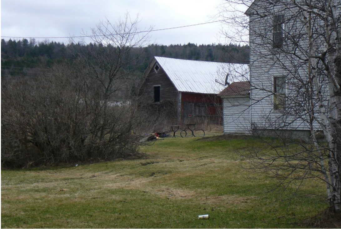
Figure 120. View northwest of gable roof barn at the former Malvern Farm location on the west side of VT Route 100.
