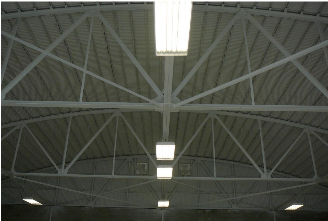
Figure 51. View of interior metal roof trusses in terminal/Esline hangar at the Caledonia County State Airport.
