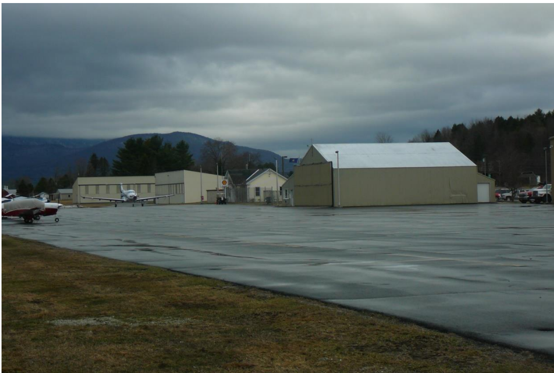
Figure 97. View southwest of southernmost buildings at the Morrisville-Stowe State Airport.
