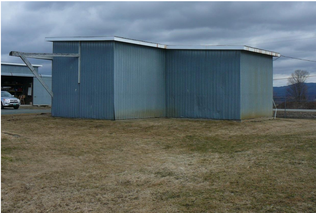
Figure 21. View northeast of rear sides of T- hangar at the Caledonia County State Airport.
