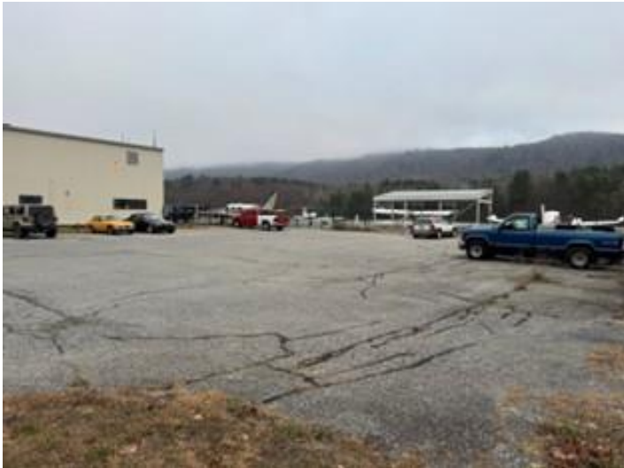
Central Terminal – looking northeast across parking lot
