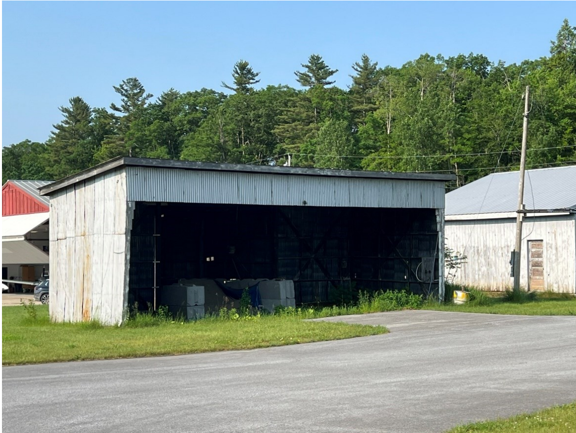
Photo 18. View of Resource 14 looking southwest.
