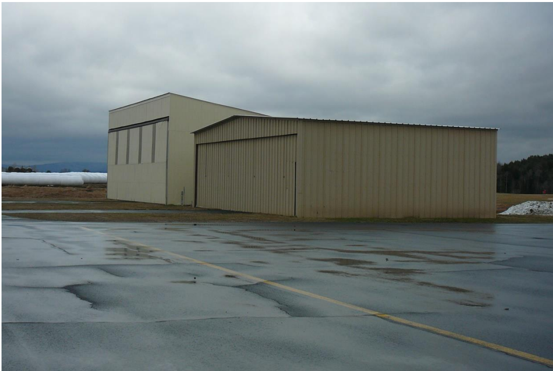
Figure 99. View northeast of hangars at the northern end of the Morrisville-Stowe State Airport.
