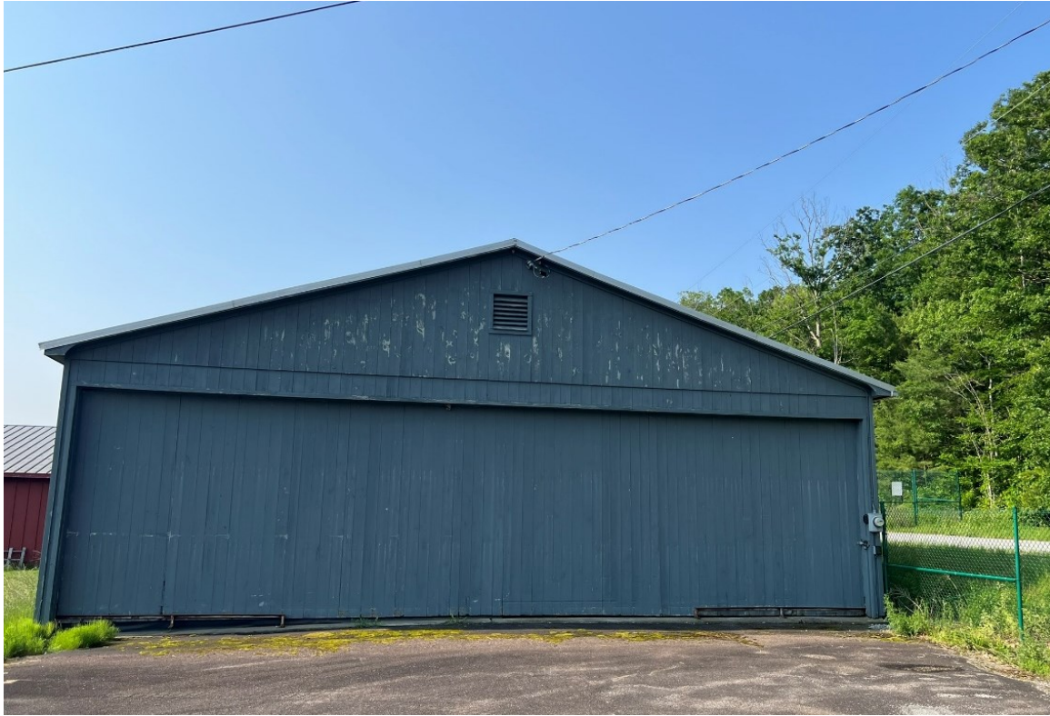
Photo 16. View of Resource 12 looking southeast.
