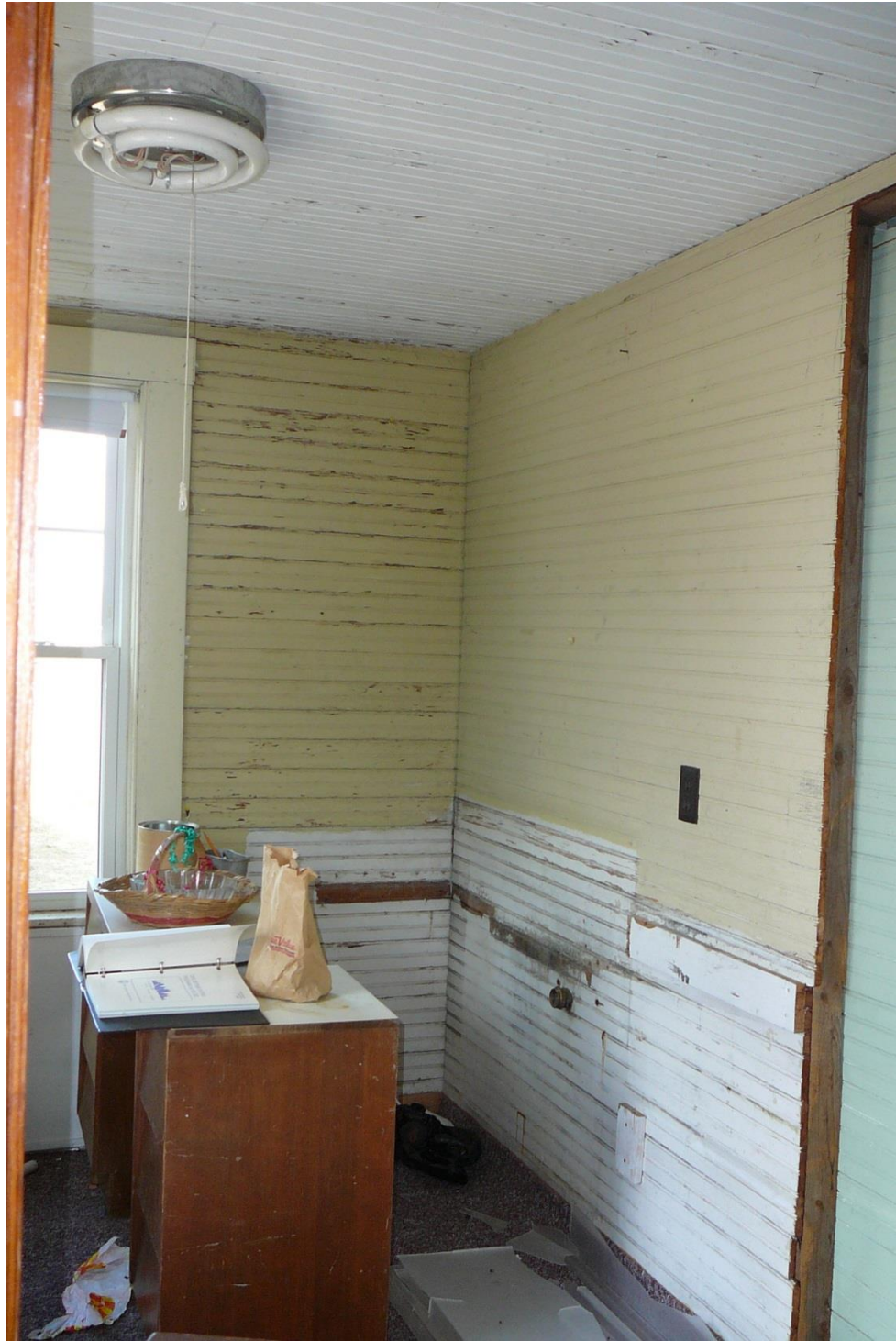
Figure 40. Small room in addition at the Pudding Hill School; note bead board wall and ceiling covering.
