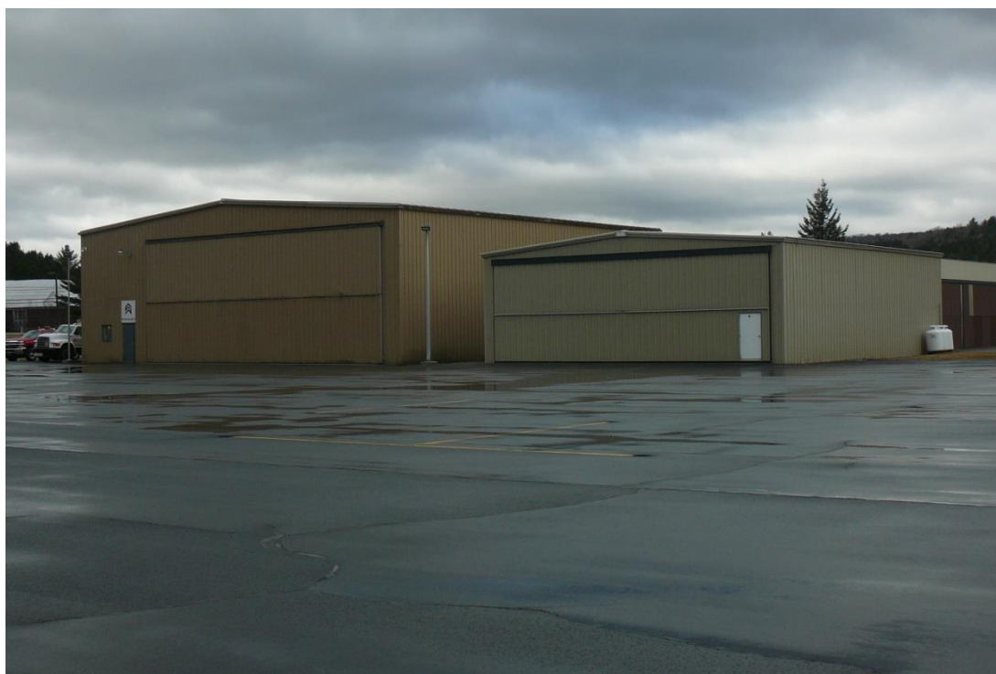
Figure 101. View southwest of hangars at the Morrisville-Stowe State Airport.
