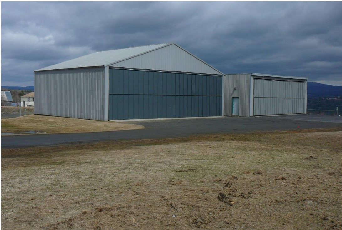
Figure 15. View southeast of the northernmost hangars at the Caledonia County State Airport.
