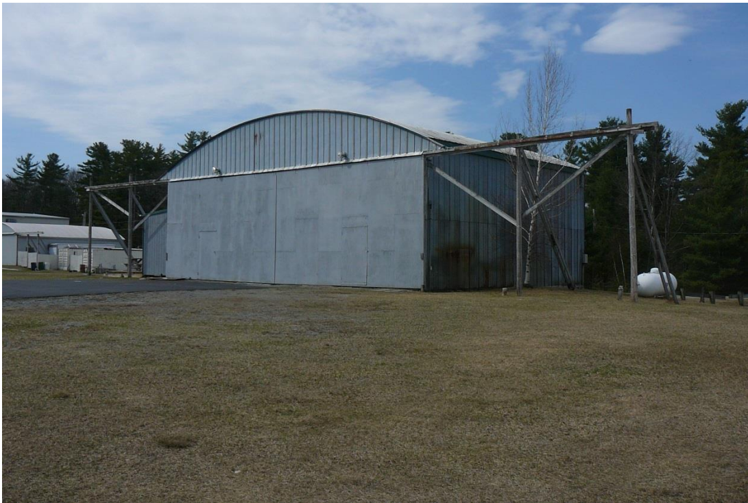
Figure 77. View southwest of arched roof hangar at the Middlebury State Airport.
