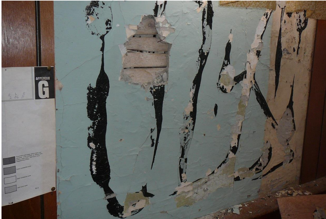
Figure 41. Exposed split plaster and lath wall at the Pudding Hill School.
