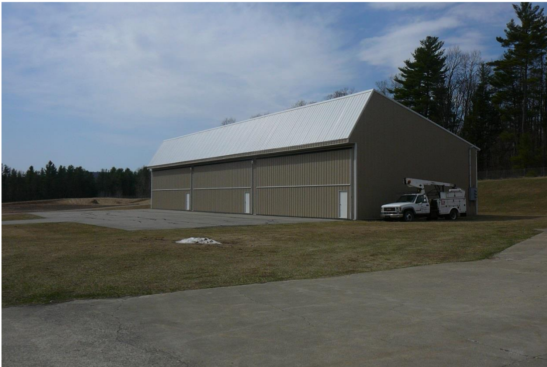
Figure 85. View southwest of southernmost hangar at the Middlebury State Airport.
