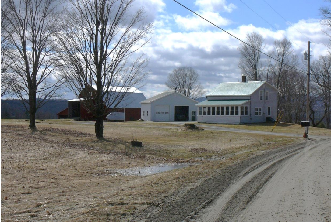
Figure 60. View southwest of the former historic Parker farm complex on the south side of Airport Road.
