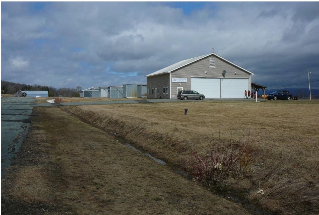
Figure 11. View northeast of buildings at the Caledonia County State Airport.
