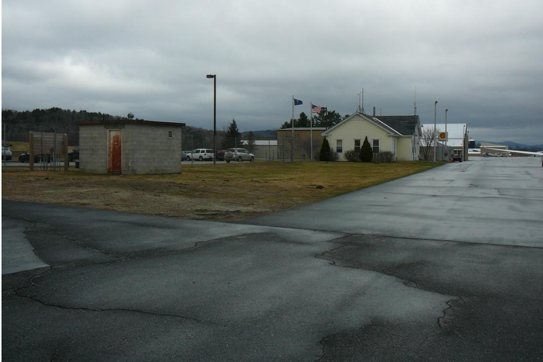
Figure 96. View northwest of buildings at the Morrisville-Stowe State Airport.
