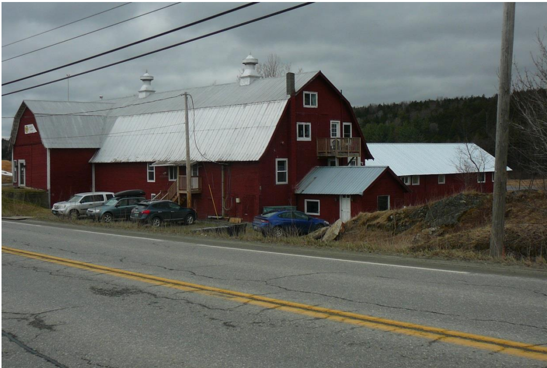
Figure 123. View northeast of barns across from the former Webster/Chaffee house, on the east side of VT Route 100.
