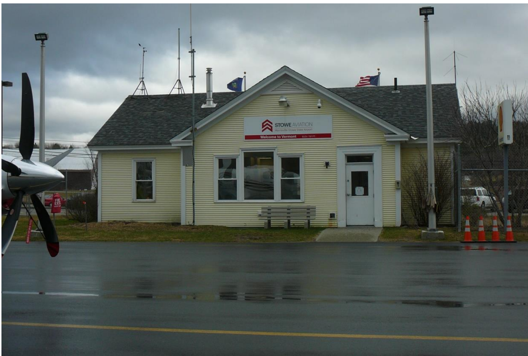
Figure 103. View west of terminal at the Morrisville-Stowe State Airport.
