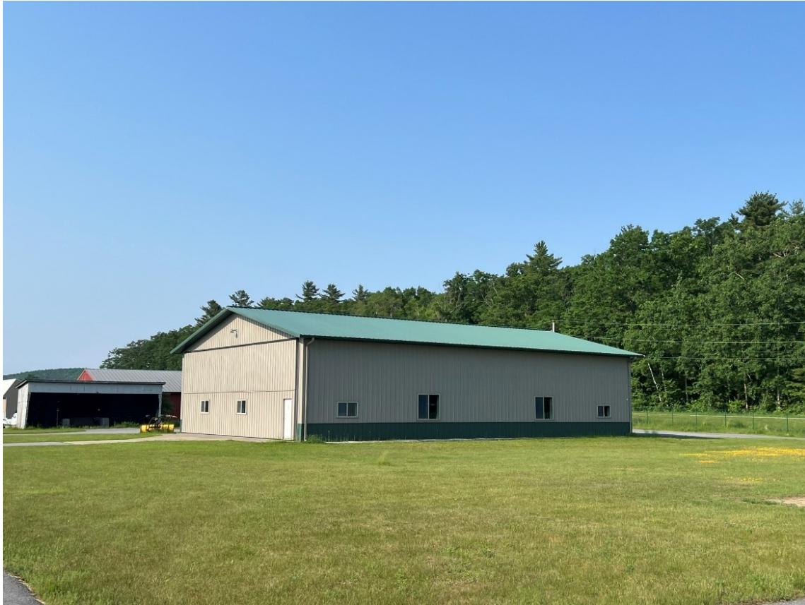
Photo 15. View of Resource 11 looking southwest.
