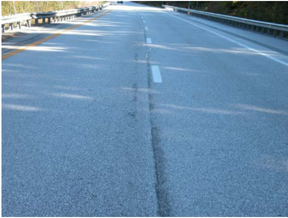
Figure 5 - Overview of Cracking in ATPB
