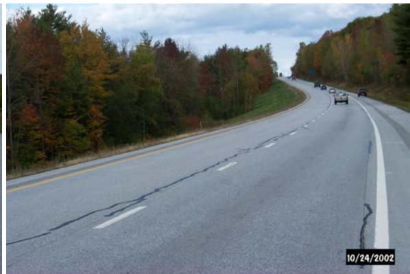
Figure 3- ATPB Site (MM 109.25) (note paving joints and sealed crack locations)
