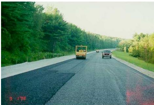
Figure 1 - Application of ATPB
