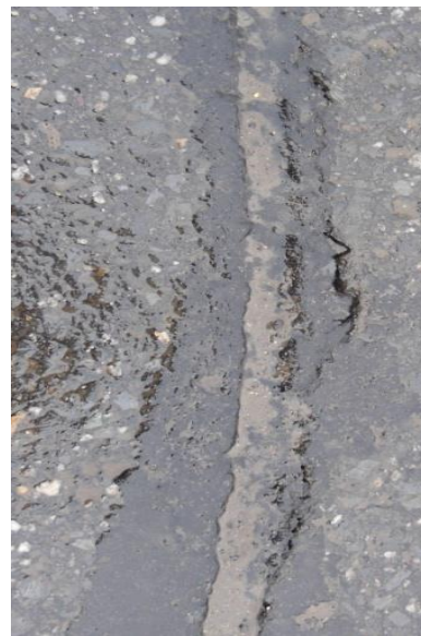
Figure 11: Spalling distress in test site 12 in Type IV section.
