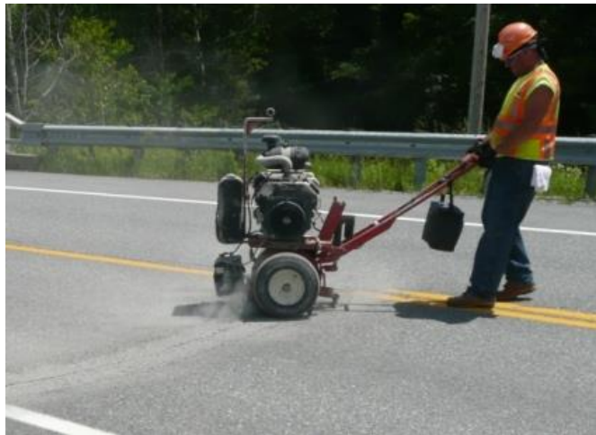
Figure 3: Typical routing operation.
