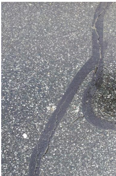
Figure 10: Adhesion loss in transverse crack in test site 7 in the Type II section.
