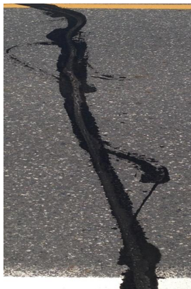
Figure 7: Transverse crack in test site 12 in the Type IV section.
