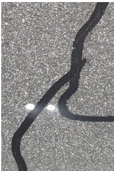
Figure 6: Transverse crack in test site 7 in the Type II section.
