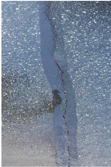
Figure 8: Adhesion loss in transverse crack in test site 2 in Extend-Pave section.
