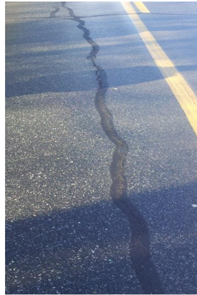
Figure 9: Longitudinal crack in test site 3 in Extend-Pave section.
