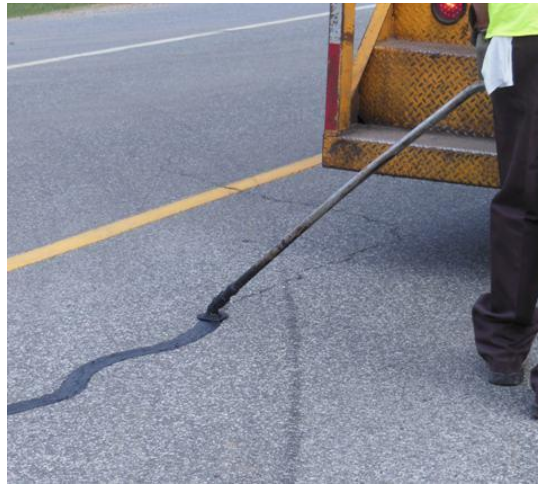
Figure 2: Blow and go crackfilling.
