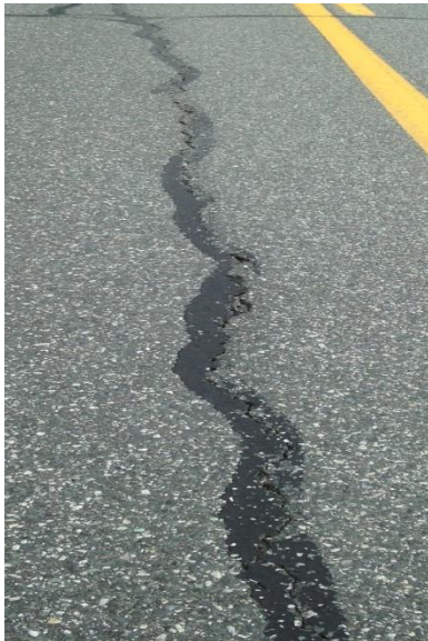
Figure 12: Adhesion distress in longitudinal crack in test site 3 in Extendo-Pave section.
