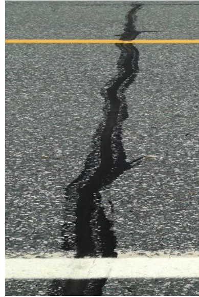
Figure 15: Transverse crack in test site 12 in Type IV section.
