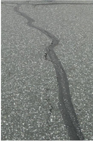
Figure 14: Adhesion distress in longitudinal crack in test site 5 in Type II section.
