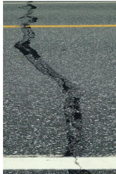
Figure 13: Adhesion distress and wearing in transverse crack in test site 4 in Extendo-Pave section.
