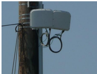
Figure 10: Connecting Wire to Sensor.
