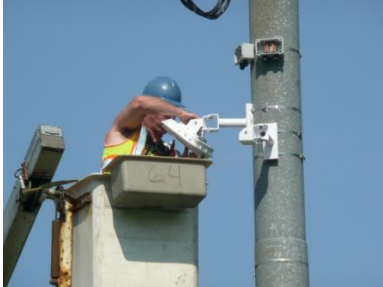
Figure 6: Anchoring Sensor.
