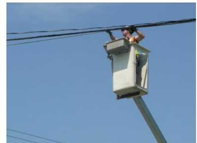
Figure 11: Running the Wire Across Intersection.
