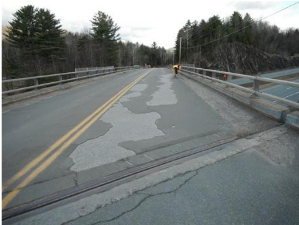
Figure 1. Condition of the previous overlay (unknown product) in 2012.
