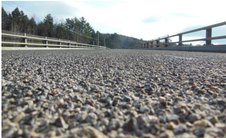
Figure 5. Surface texture of Flexogrid.
