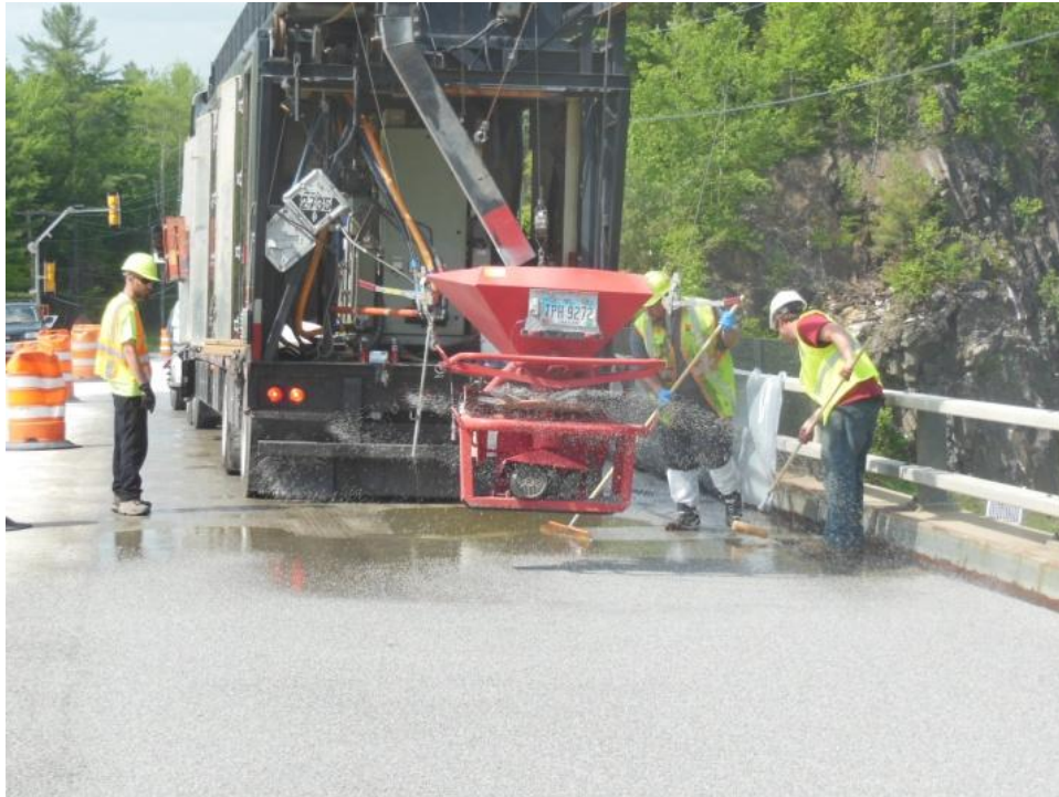
Figure 3. Installation of Flexogrid. Epoxy has been squeegeed on and the aggregate is being spread on the surface.
