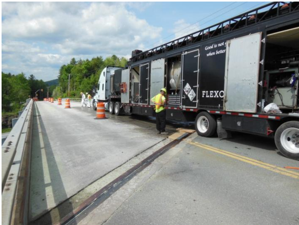
Figure 2. Poly-Carb installation vehicle, and the prepared condition of the concrete bridge deck.
