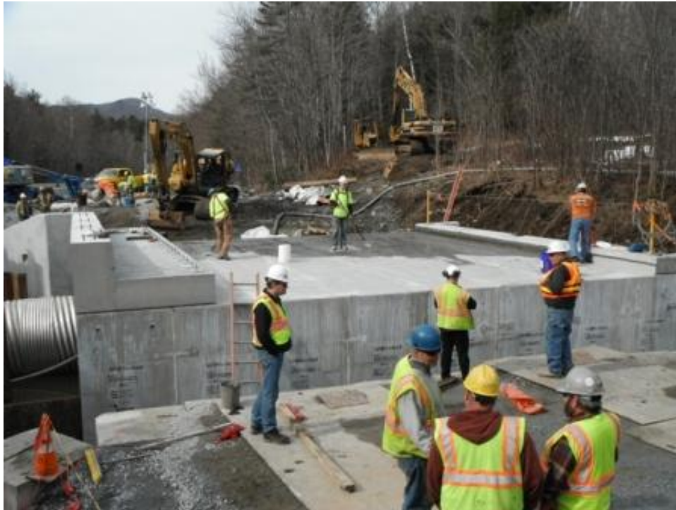
Figure 1 Installation of the BDM system, application of the primer
