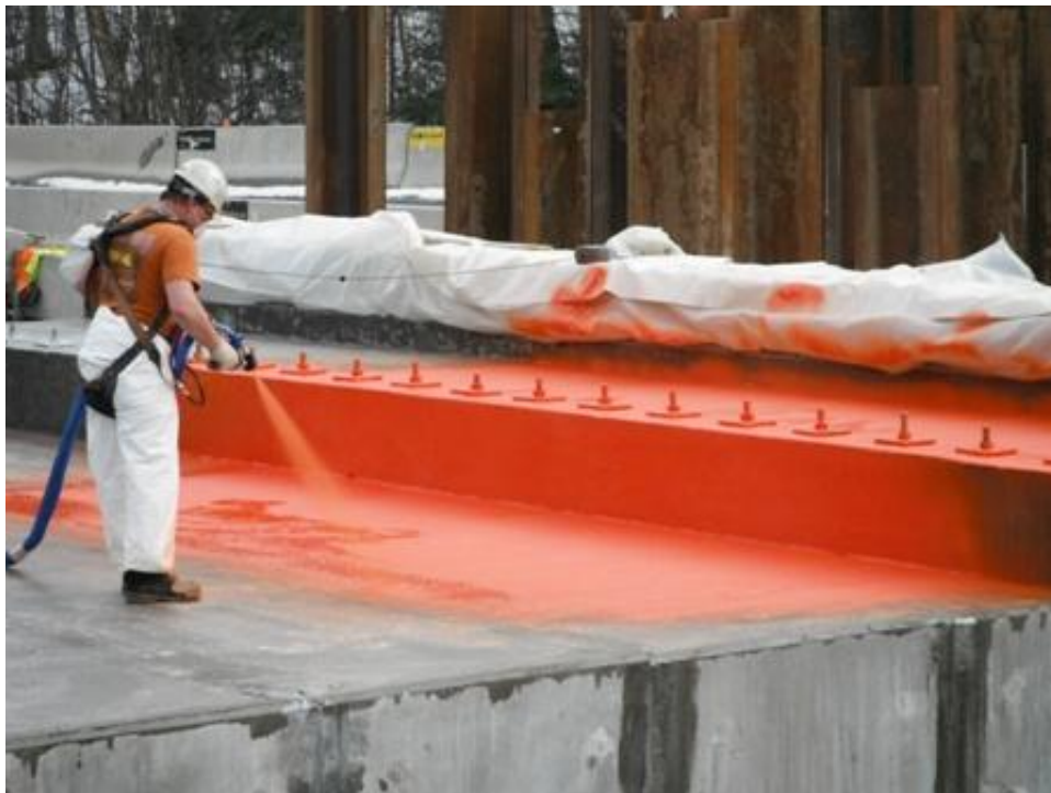
Figure 2 Spraying of the membrane
