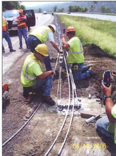
Figure 1 – Brifen Wire Rope Installation
