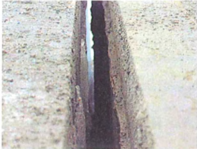
Photo -1 Looking west
