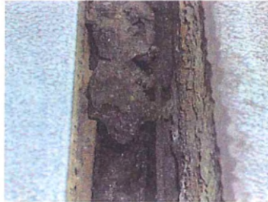
Photo -2 Looking west
