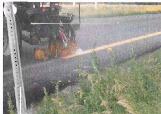
Figure 3- Yellow Edge line being applied (MM 0.55 WB)
