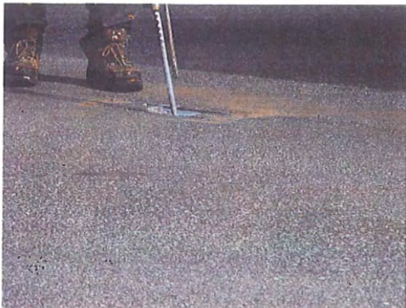
Figure 3 – Applying epoxy
