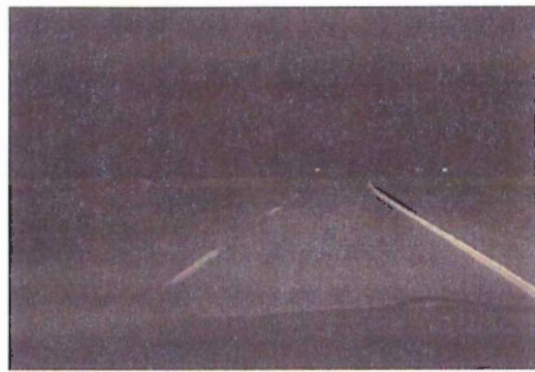
Thermoplastic on skip lines (Aug. 3, 2004)
