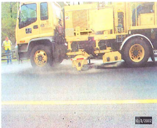
Grinding of Pavement
