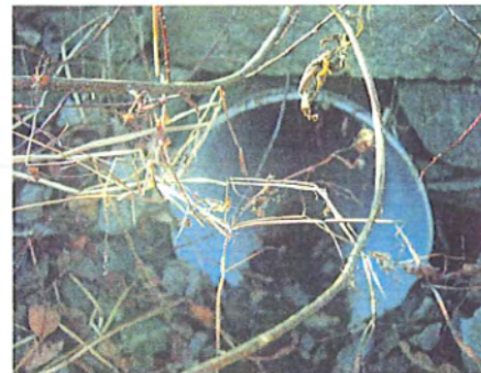
450mm Pipe Outlet - Stone Headwall (East End) Front View
