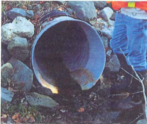
600mm Pipe Inlet (West End) Front View
