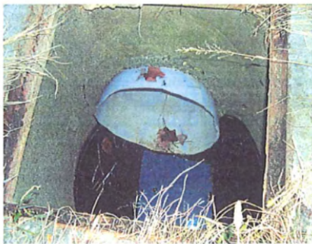
450mm Pipe Catch Basin (West End) Top View with Grate removed
