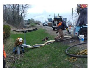
To prepare the product for installation, steam was applied to the liner for approximately 4 hours by covering the entire spool with tarps and injecting the steam within the tarps. The time needed to soften the liner depends on the length and diameter of the liner as well as the ambient temperature. Once the liner was sufficiently malleable it was pulled through the existing pipe with a winch.
