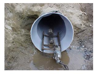
camera which can be fed through the entire length of the culvert. The entire process of lining one culvert took one working day to complete.
