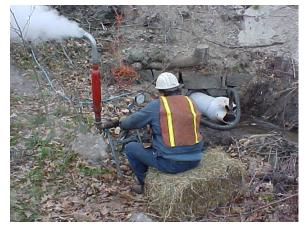
According to the manufacturer's documentation the pressure within the liner is never to exceed 12 PSI. For this installation pressure was brought to 5 PSI. Once the liner has taken the shape of the existing pipe the injection of steam is stopped and only compressed air is applied to cool the liner. The temperature of the exhaust air was brought down to 100 degrees before the pressure was released.
