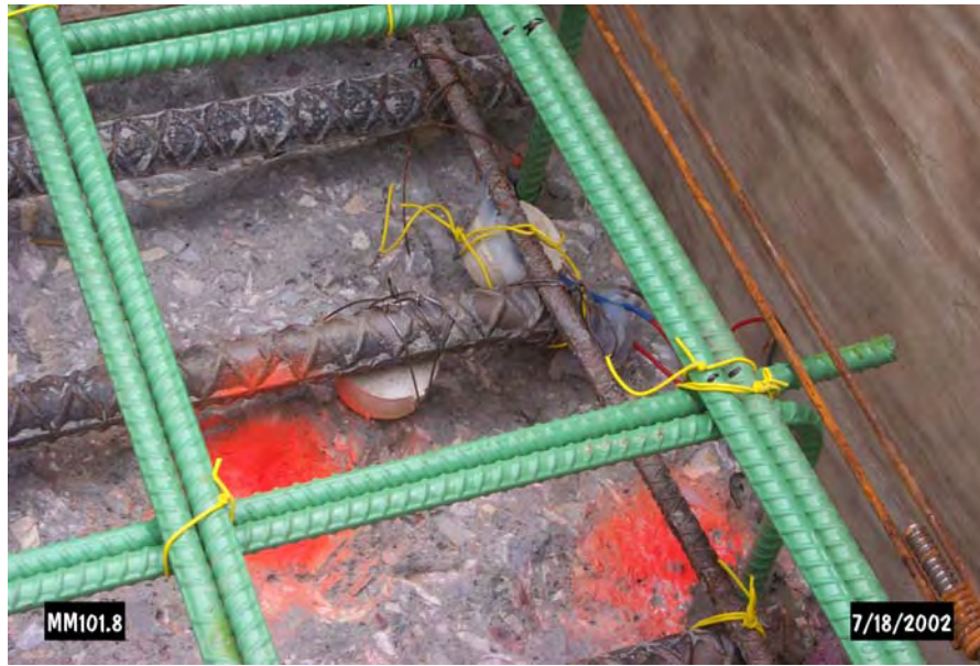
Galvashield XP Anode and Test Kit installed in the Cap of Pier 2 on Br. 48N
