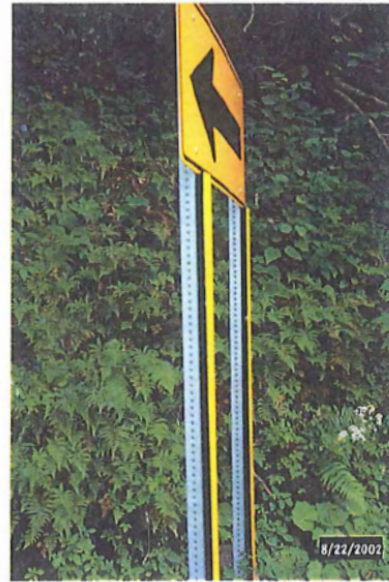
Figure 3. Ripton – Vermont Route 125 Square-Tube Posts w/ Diamond Grade Sheeting.
