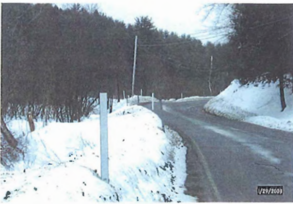
Figure 4. Chester – Vermont Route 10 U-Channel Posts w/ Diamond Grade Sheeting.
