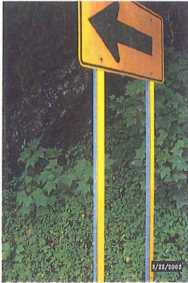
Figure 2. Ripton – Vermont Route 125 U-Channel Posts w/ Diamond Grade Sheeting.
