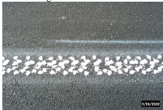
Figure 4. Detail of pavement marking material retained for evaluation.
