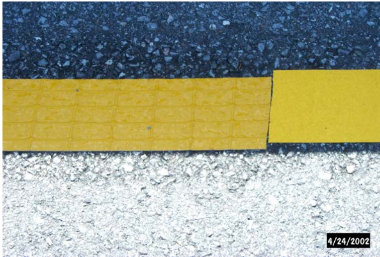
Figure 2. 3M™ Scotch-Lane™ Wet Reflective Removable Tape Series 750 adjacent to non- wet reflective temporary tape.
