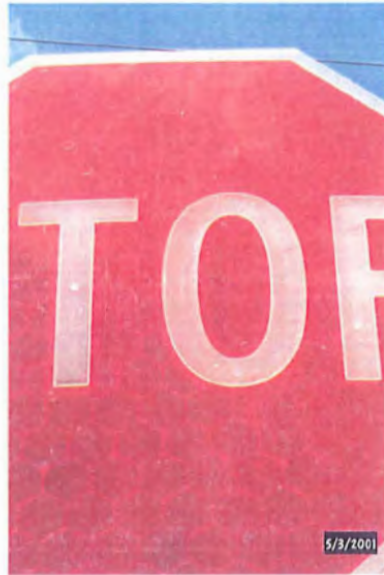
Figure 7. Marshfield – Scratches on sign face.
