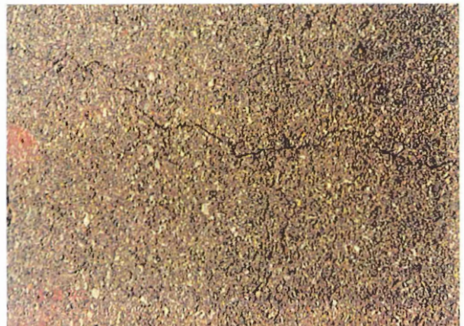
Figure 5. Development of hairline cracks. (Photo taken May, 2000)
