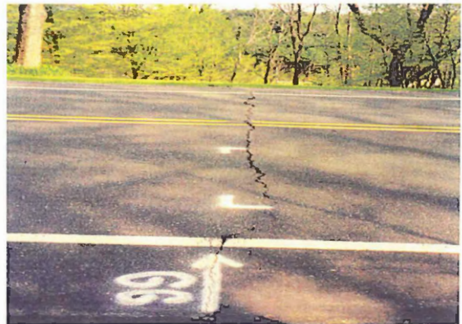
Figure 7. Full-length transverse crack, developed after 1½ years performance (9m south of material's north edge). (Photo taken May, 2000)
