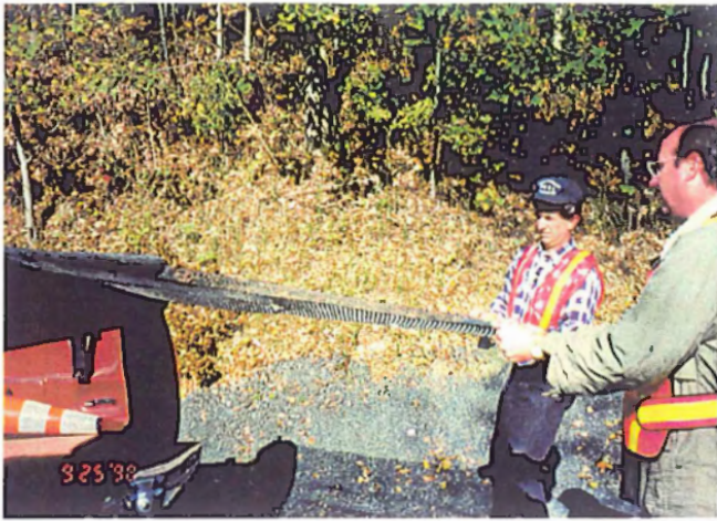
Figure 2. Installing GlasGrid® in Barnet.
