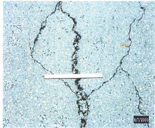
Figure 2. Formation of polygon cracks from existing longitudinal crack in westbound lane (RCB) at MM 2.33.
