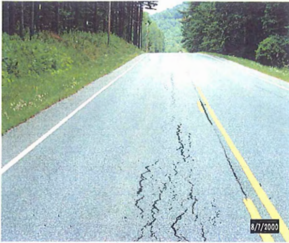
Figure 1. Distress in westbound lane treated with CaCl at MM 1.65.
