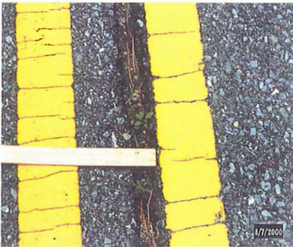
Figure 3. 25 mm centerline crack at MM 1.72.
