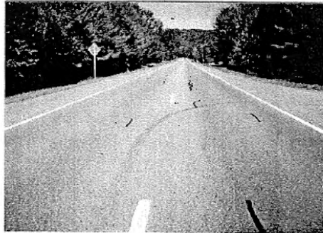
Figure 2 Cold Planed Treatment
