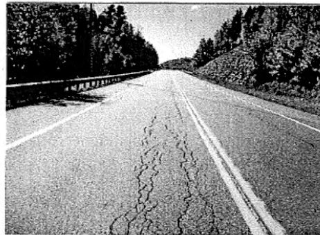
Figure 3 Cold Recycled Bituminous Pavement (CRBP)
