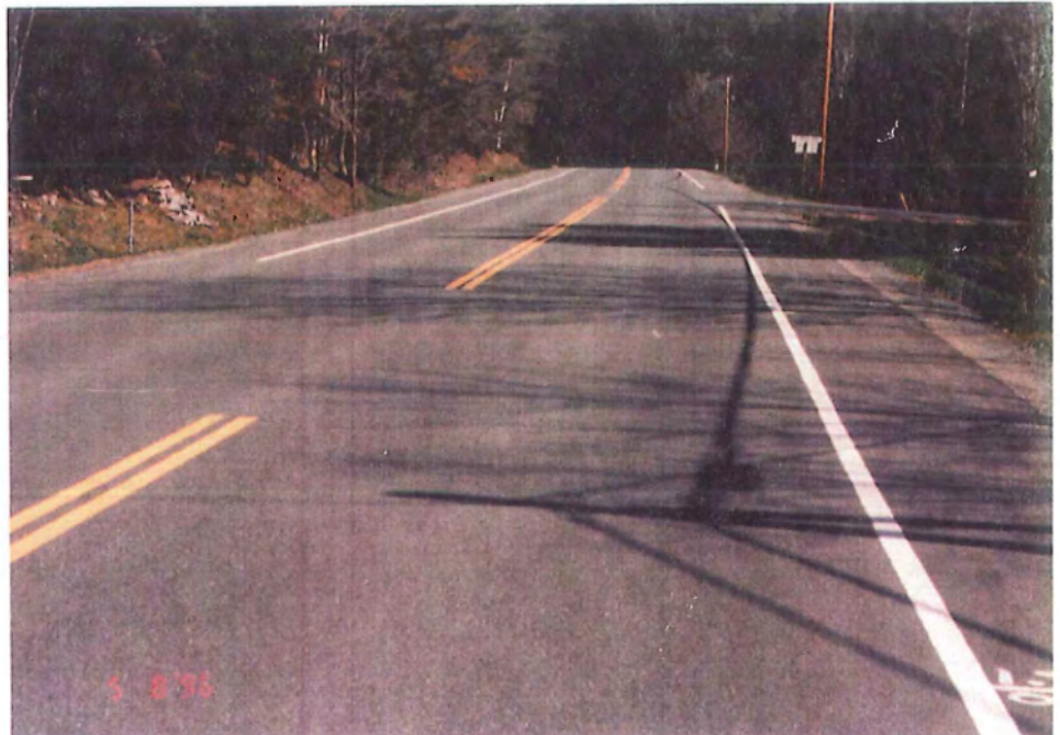
Reclaimed Base with PG 52-40 asphalt cement VT 18, Waterford, MM 1.73
