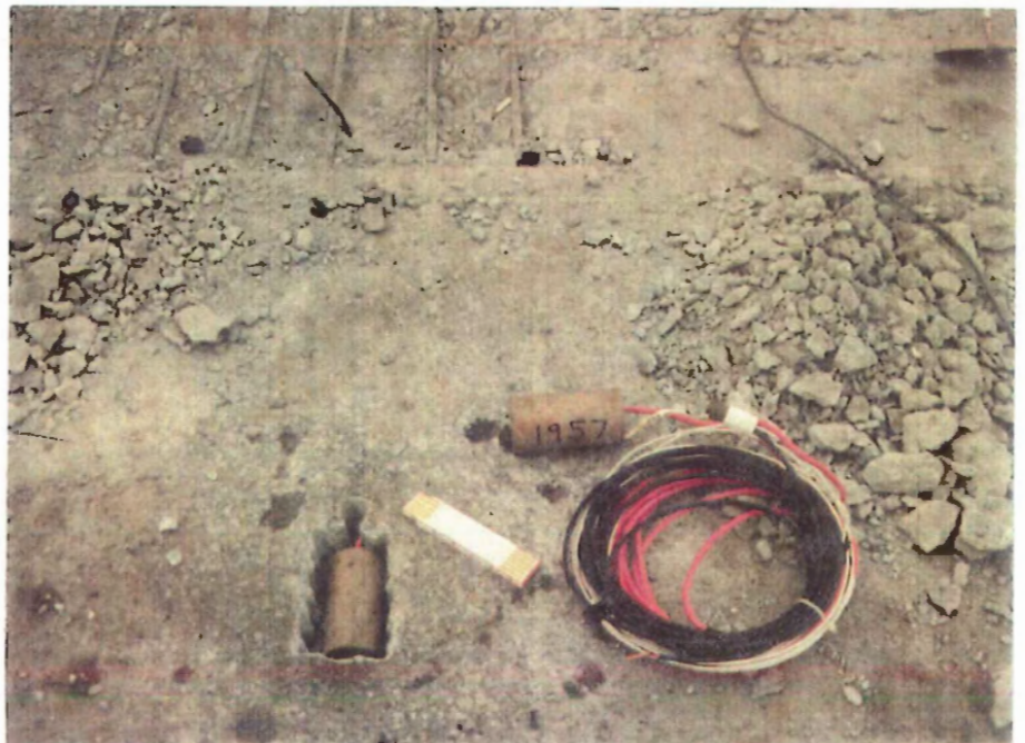
INSTALLATION OF PROBES IN BRIDGE DECK
