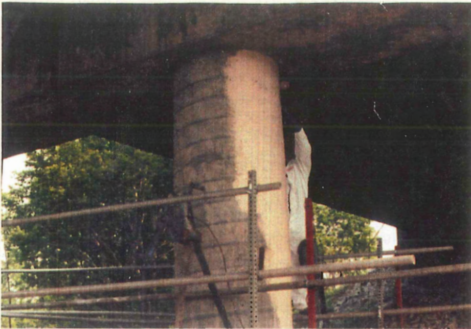
Epoxy-paint mixture was applied to repaired areas.
