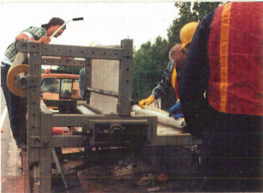
Glass Fabric was drawn through rollers and saturated with epoxy resin.
