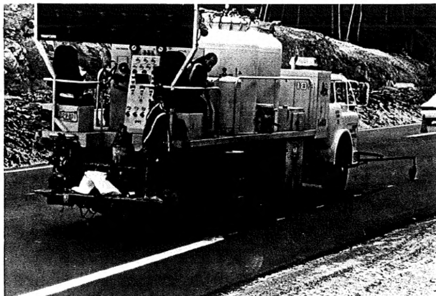
Fig. 1 Truck Mounted, Airless Spray
