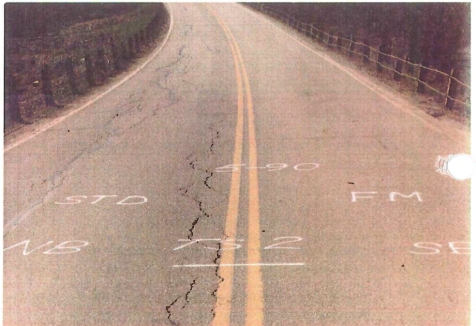
STD Mix vs FM (10 lbs/ton) Fiber Mix treatment ends in background of FM lane.
