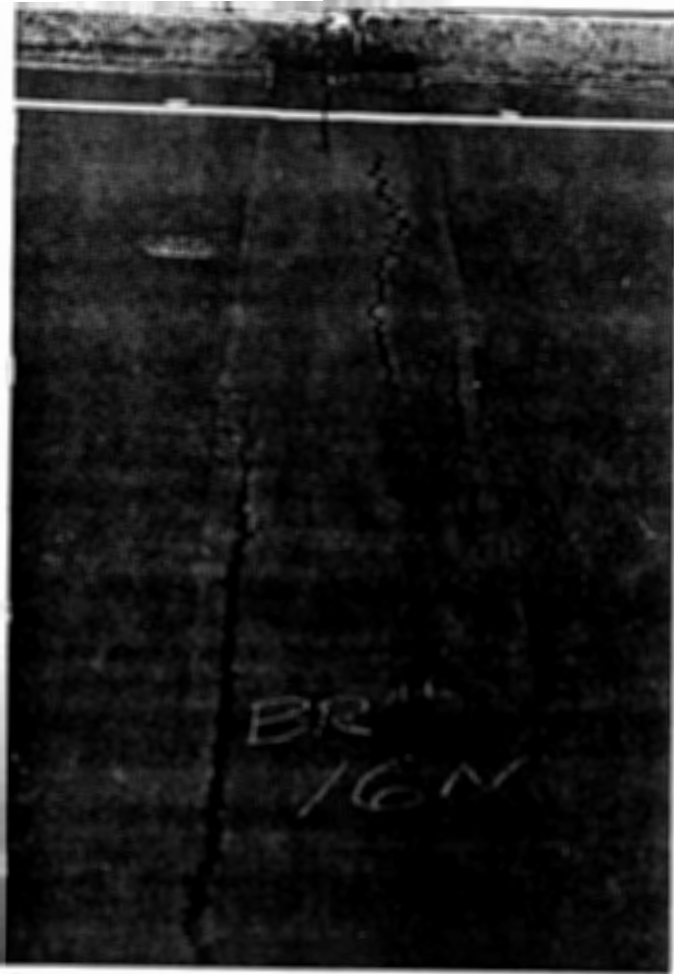
Thorma-Joint System Failure in North Joint
