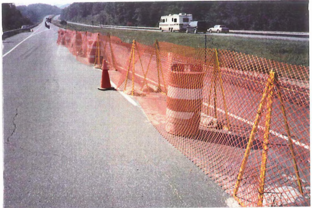
Photo 2 Installation on Porta Posts
