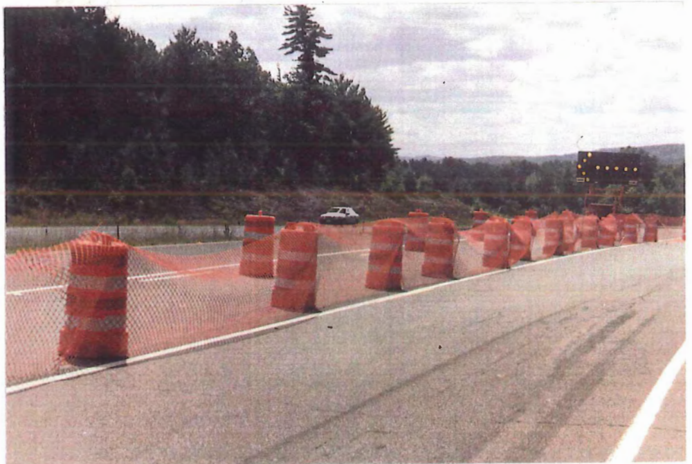
PHOTO 1. Installation on Drums
