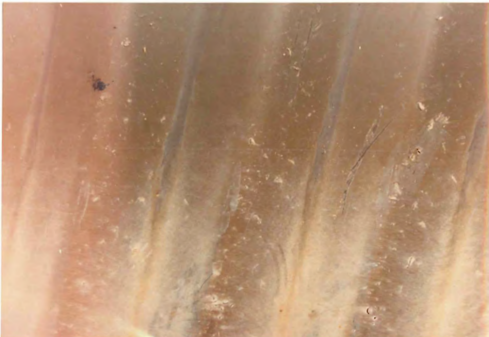
Note nicks in coating on up stream side of corrugations
