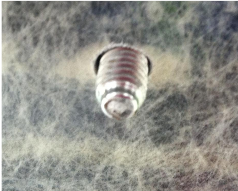
Figure 10 Swedge Bolt Anchored.
