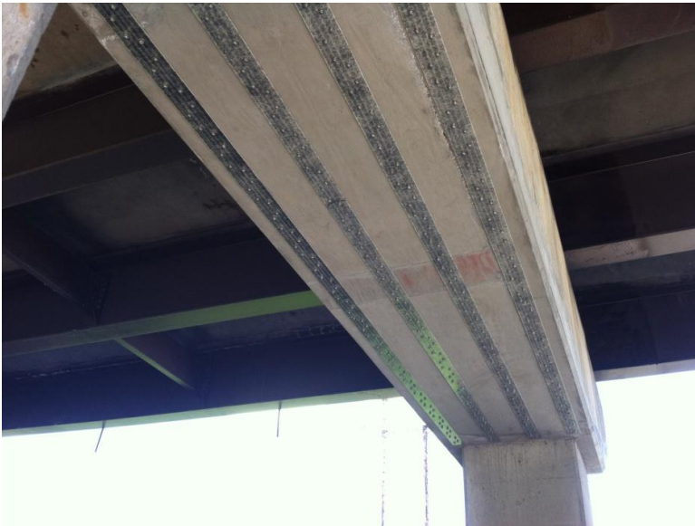
Figure 8 Completed FRP Installation
