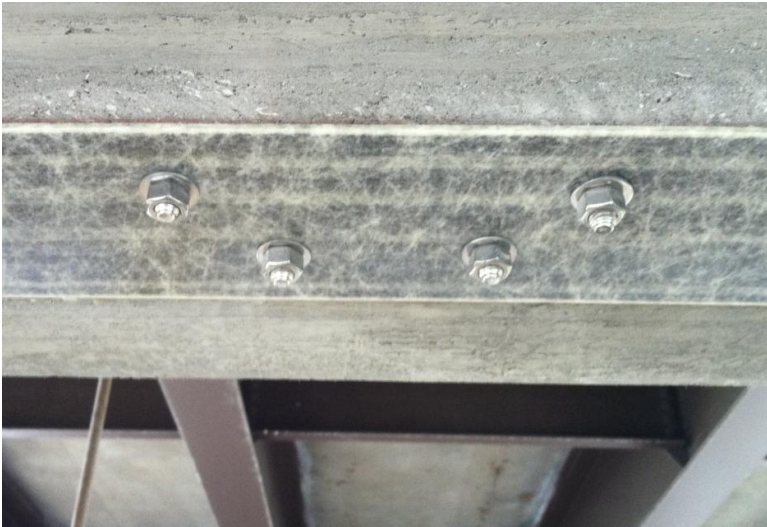
Figure 7 Completed Pattern of Bolts.
