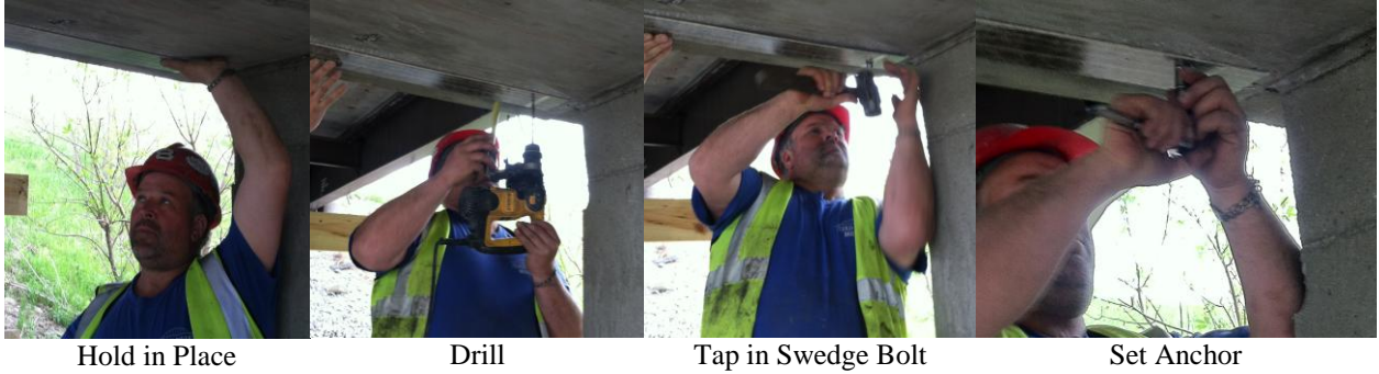
Figure 6 Sequence of Installing FRP Strips.
