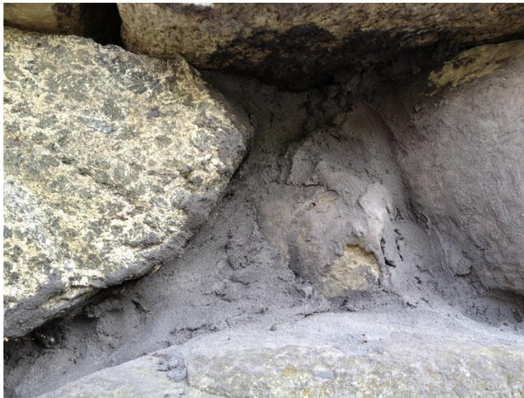
Figure 14 Up-close view of stone pointing and mortar work (VTrans 2013)
