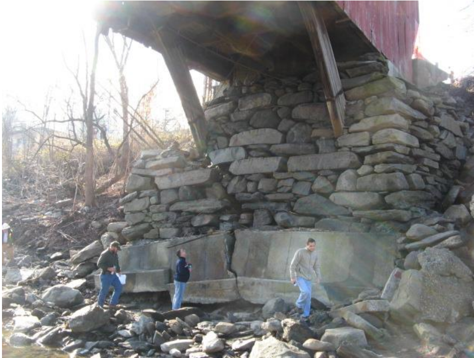
Figure 8 Westerly abutment partially collapsed (VTrans 2011)
