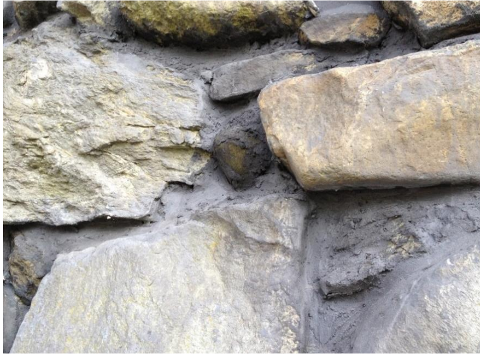
Figure 15 Completed mortar work (VTrans 2013)
