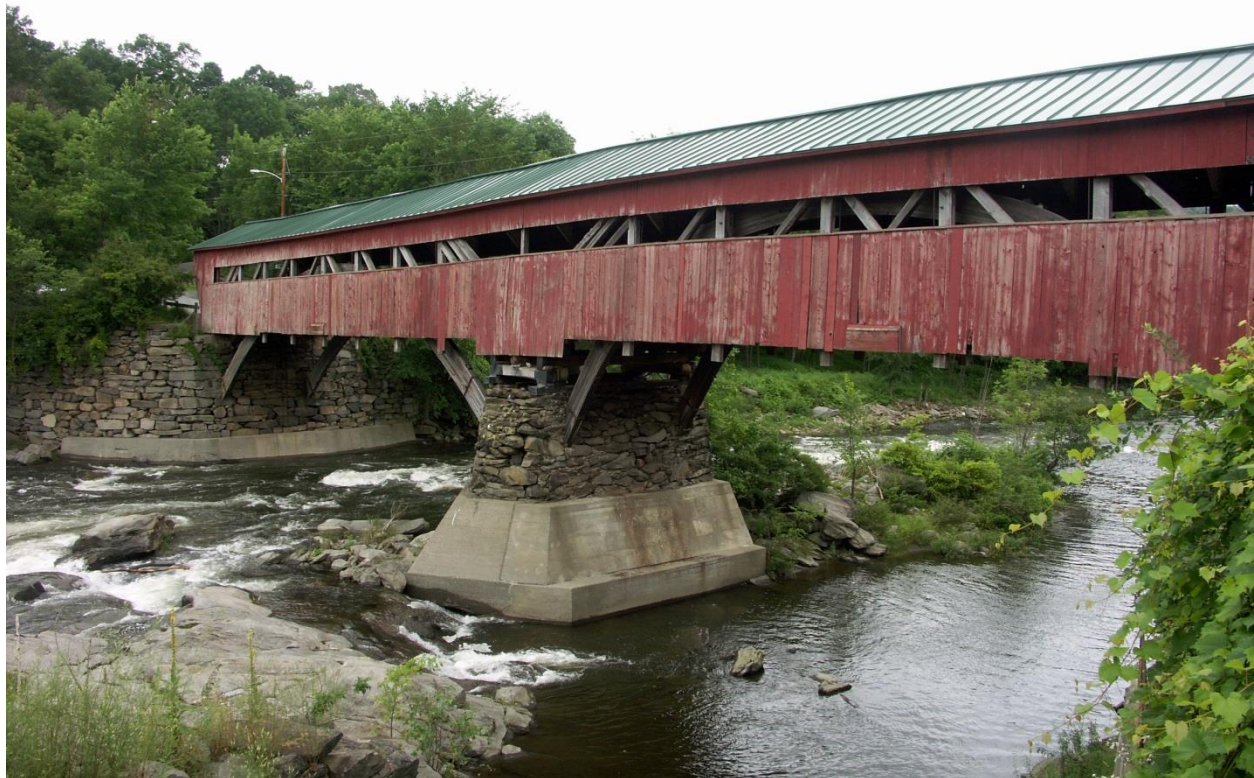
Figure 2 The Taftsville Covered Bridge in 2006 showing the Pier and Abutment that were preserved ( cmh2315fl )
