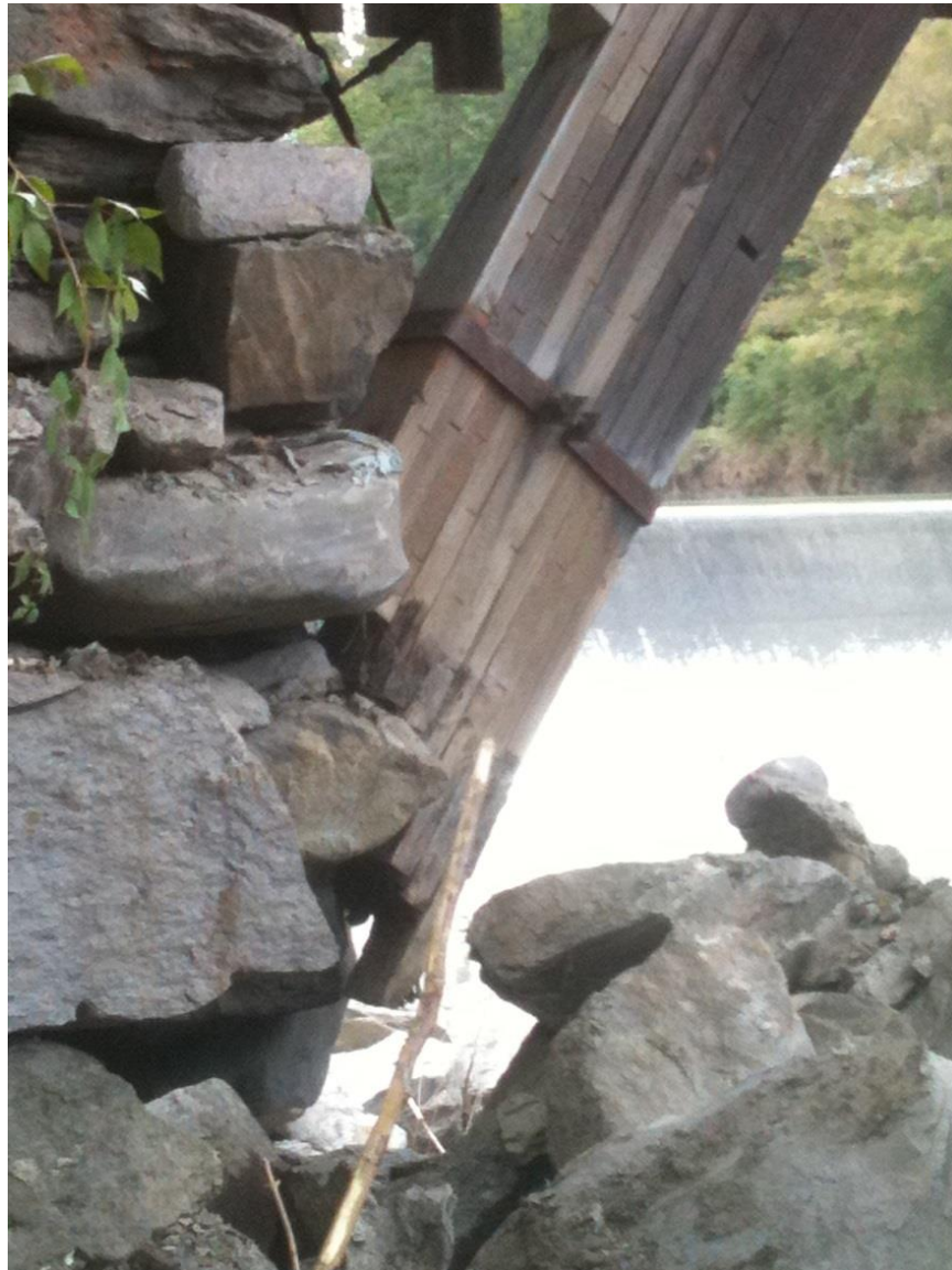
Figure 10 Downstream westerly arch dislodged from abutment (VTrans 2011)
