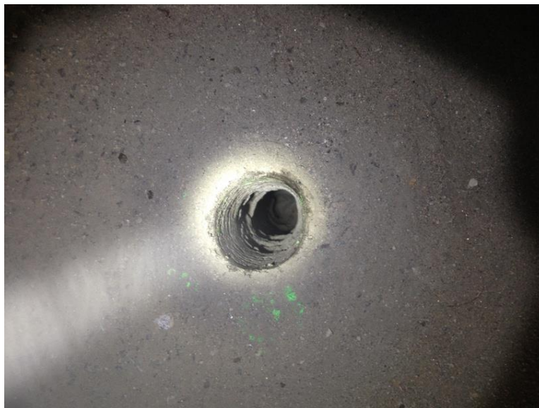
Figure 5: Drilled Injection Hole (2.5 inches x 20 feet)
