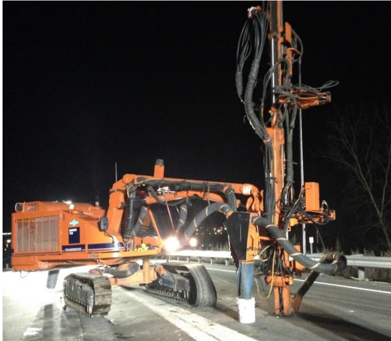
Figure 4: Tamrock 700 Drill Rig – Drilling 2.5-inch Injection Holes.
