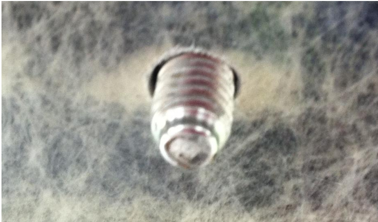
Figure 17 Swedge Bolt Anchored (VTrans 2014)
