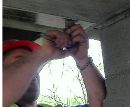
Set Anchor with ratcheting socket wrench
