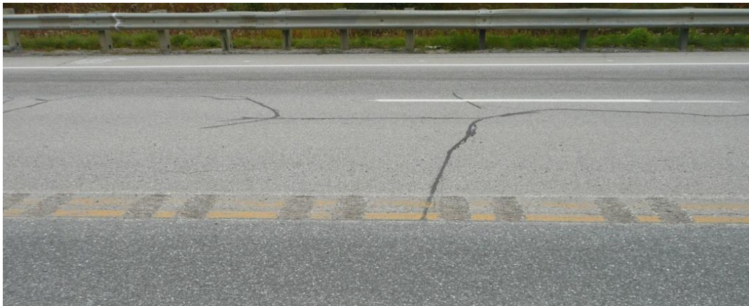
Figure 8: Rumble stripes after milling and sweeping.
