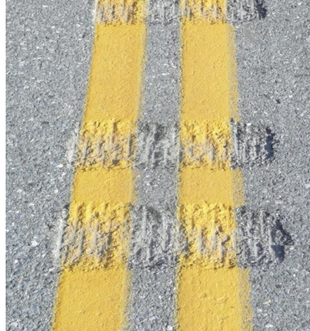
Figure 9: Centerline rumble stripes approximately one month after installation in Mendon, VT.
