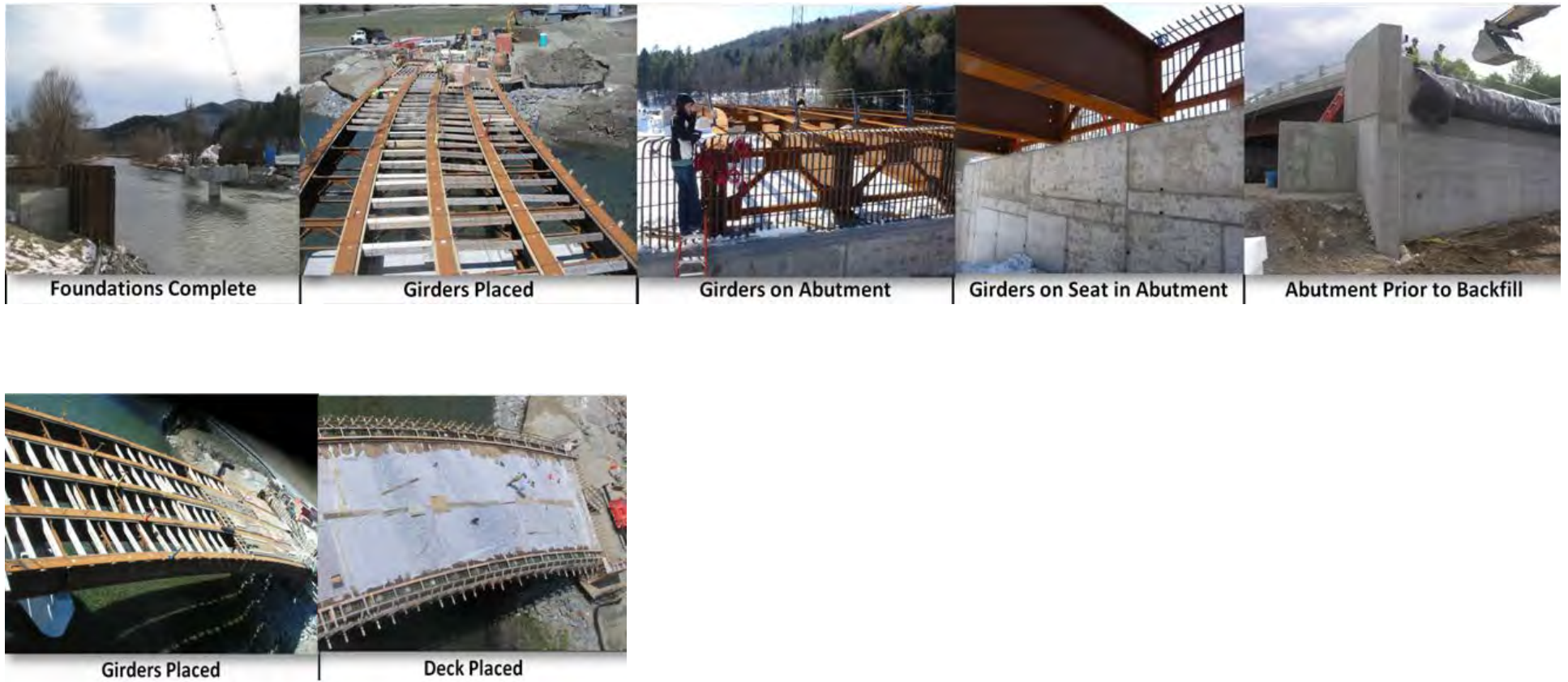
Figure C-0-6: Stockbridge Construction
