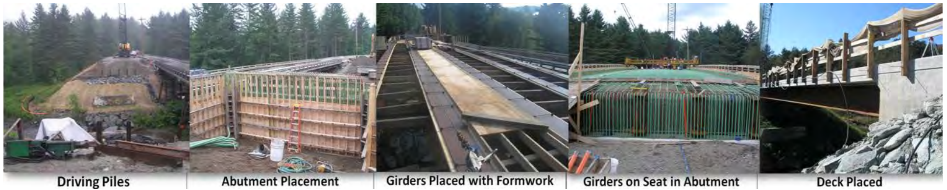
Figure C-0-4: Middlesex Bridge Construction
