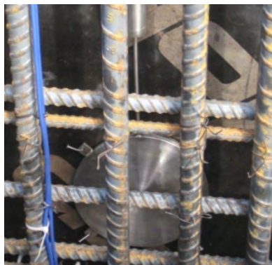
Figure 3-43: Earth Pressure Cell Installation
