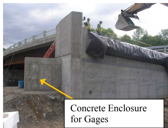
Figure 3-46: Displacement Transducer Enclosure
