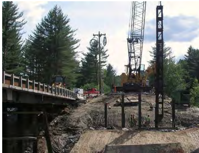
Figure 7-1: Pile Driving at the Middlesex Bridge
