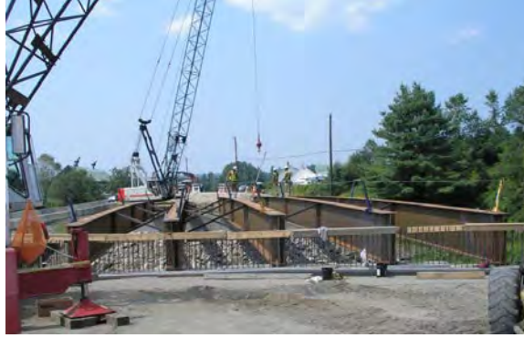
Figure 7-2: Girders Placed at the East Montpelier Bridge
