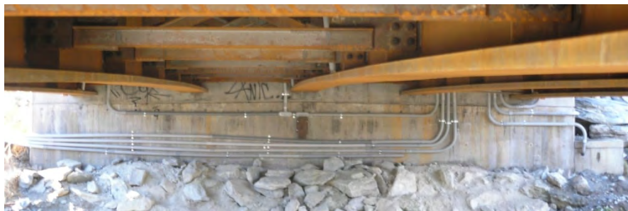
Figure 3-2: Cable Routing on the Abutment
