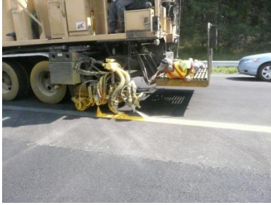
Figure 2: Spray Application of Northbound Yellow Line Delineation
