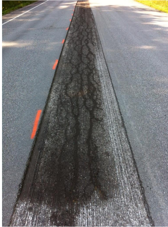
Figure 4 Roadway centerline after milling.
