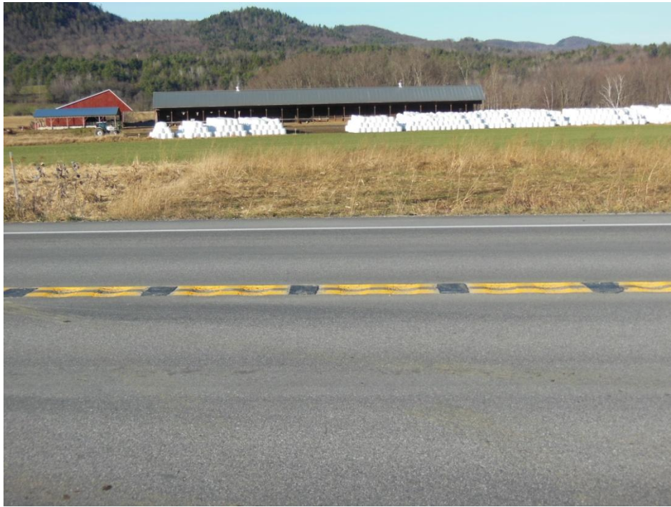
Figure 3 Initial Repair Pattern - Patched every third rumble to approximate standard.
