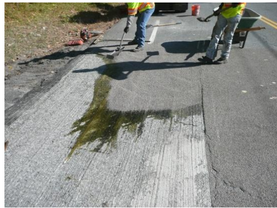
Figure 9: Spreading the aggregate
