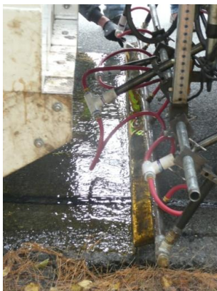
Figure 2: Epoxy truck application
