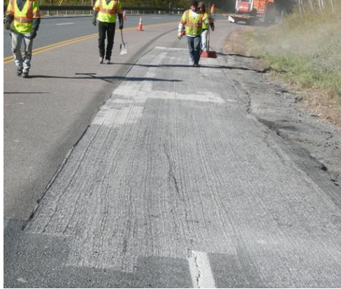
Figure 6: Repair area, after grinding and sweeping
