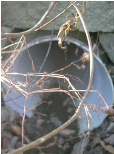
Figure 5: 18-inch pipe outlet, 2004
