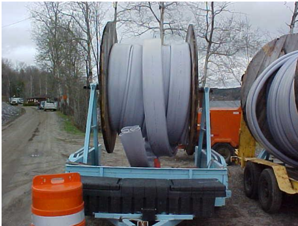
Figure 1 Spooled Ultraliner on the project site.
