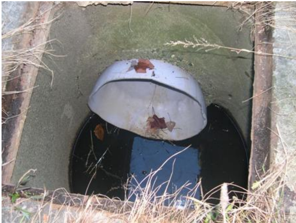
Figure 9: Photograph of the inlet of the 18-inch liner in 2004.
