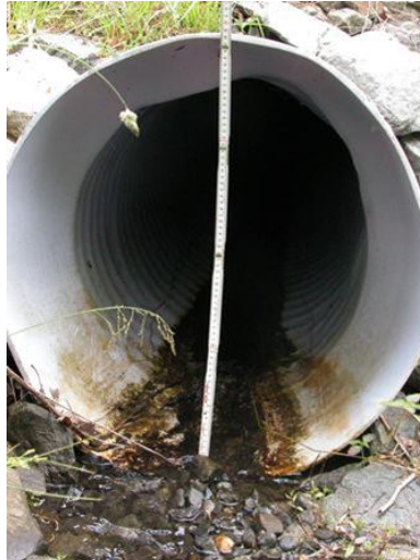
Figure 3: Inlet of 24-inch pipe, 2007
