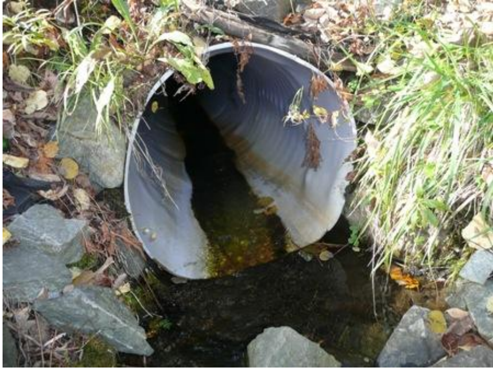
Figure 8: Photograph of the outlet of the 24-inch liner in 2010.
