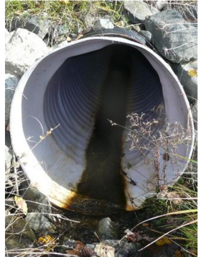
Figure 4: Inlet of 24-inch pipe, 2010
