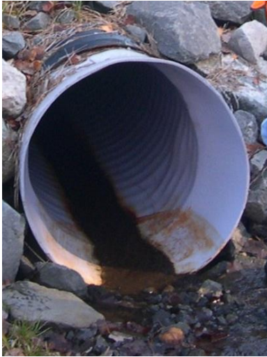
Figure 2: Inlet of 24-inch pipe, 2004
