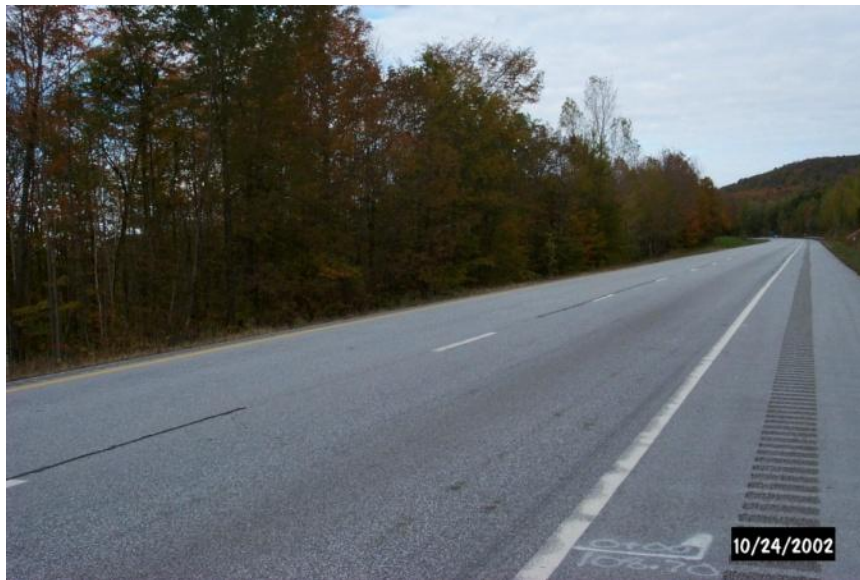
Figure 4 Typical Control Site (MM 108.70)
