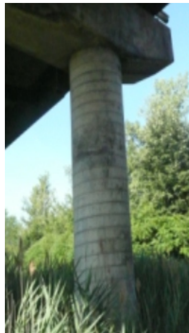
Figure 11: Column #3 under pier #2, 2010 not treated with TYFO S Fibrwrap
