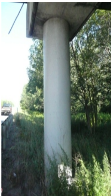
Figure 10: Column #3 under pier #1, 2010 treated with TYFO S Fibrwrap
