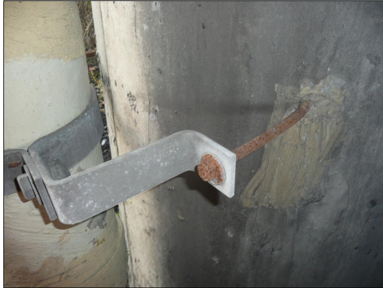
Figure 2 - Deformed Bolt
