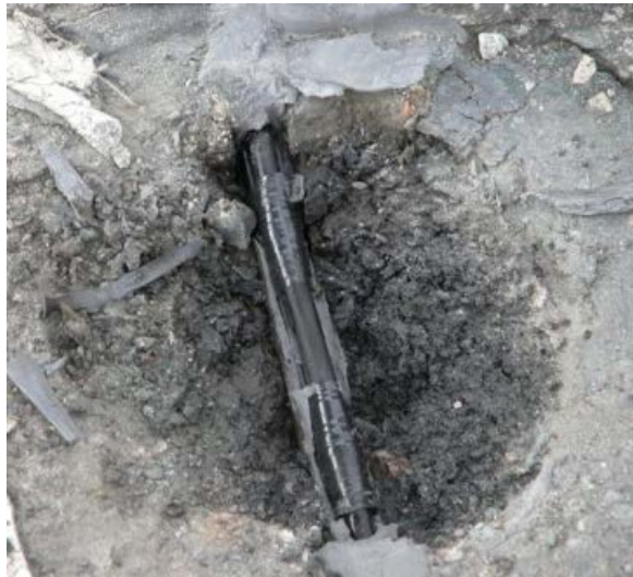
FIGURE 3 Holes after LED removal.
