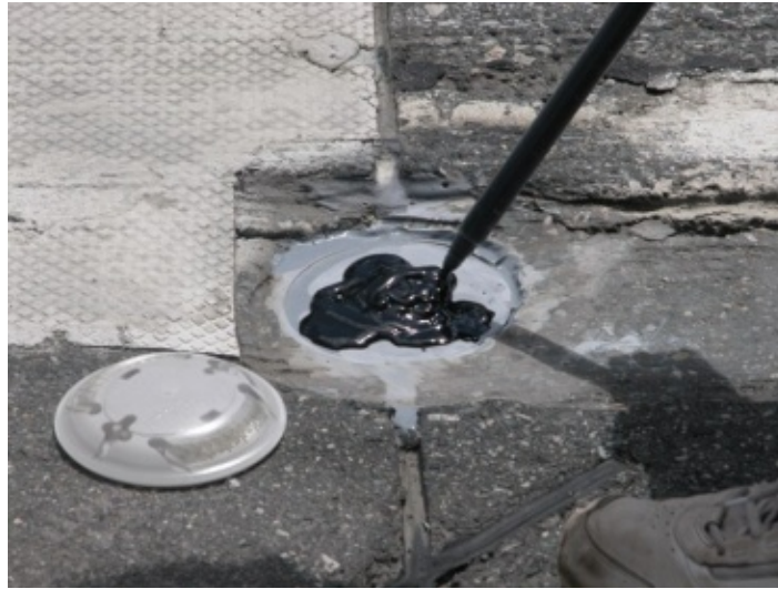
FIGURE 6 Epoxy application.
