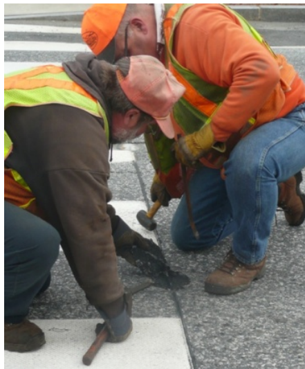
FIGURE 9 Removing Smartstud™ LEDs.
