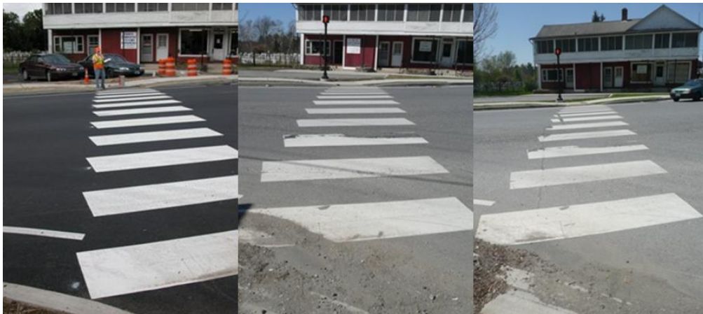
Figure 3. Progressive wear characteristics of test site 1, from left to right, at 0, 8, and 19 months post construction.
