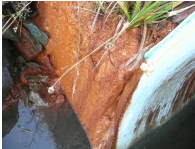
Figure 6. Photograph of the slimy material present on the outlet headwall.
