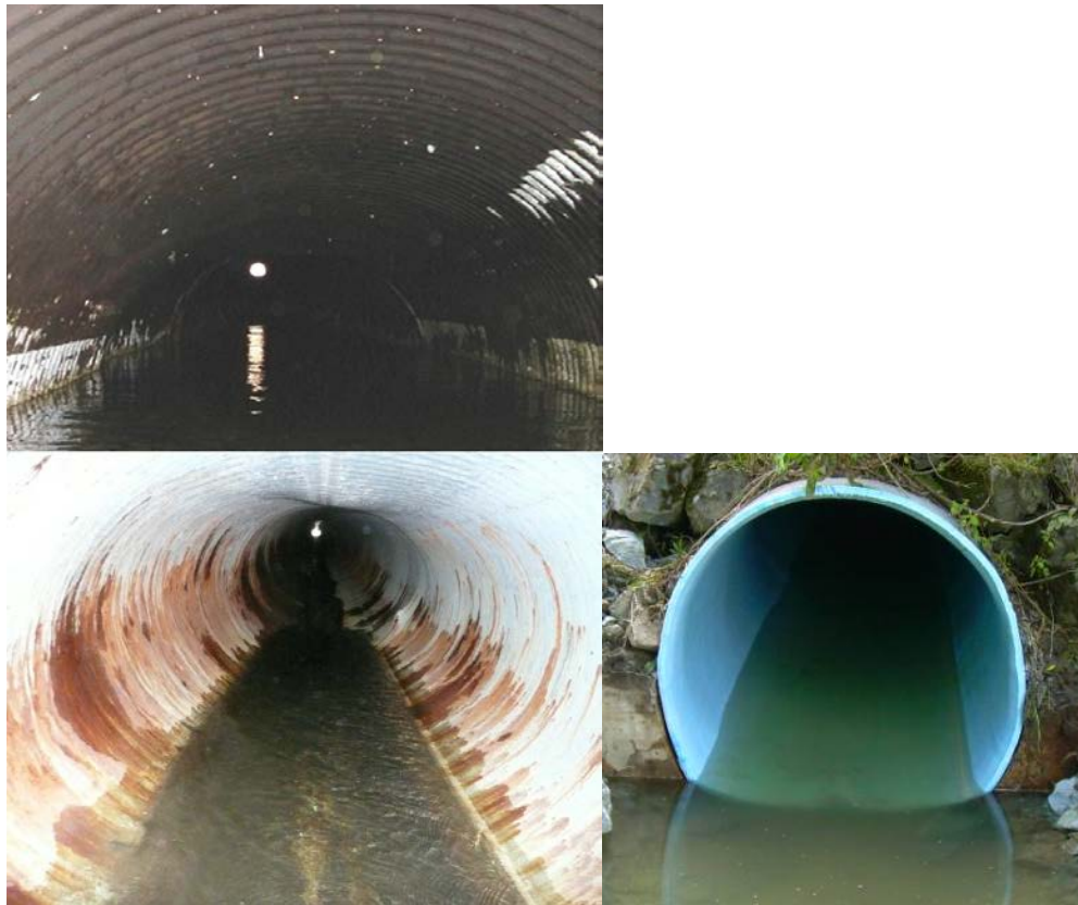
Figure 2. Condition of the outlet of the culvert at preconstruction (top), post-construction (bottom right), and present (bottom left).
