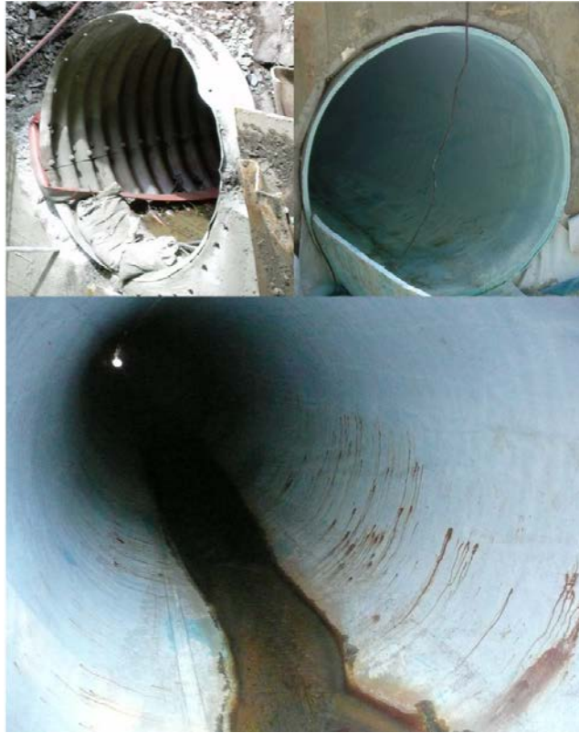
Figure 1. Condition of the inlet of the culvert (clockwise from top left), preconstruction, post-construction, and present.
