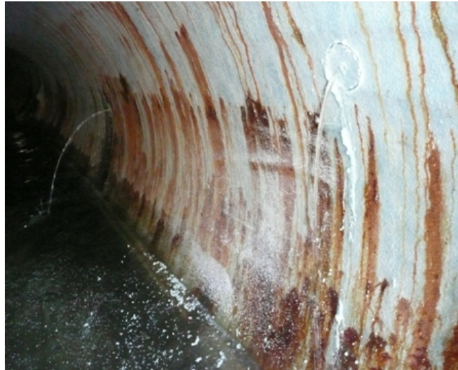
Figure 3. Water flowing into the culvert at sample 2 (far) and sample 4 (near).
