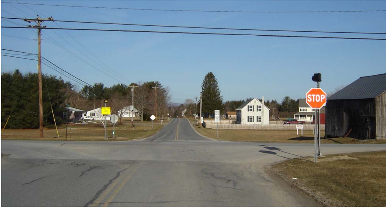
Figure 10: Installed beacon system (view is from South Street).
