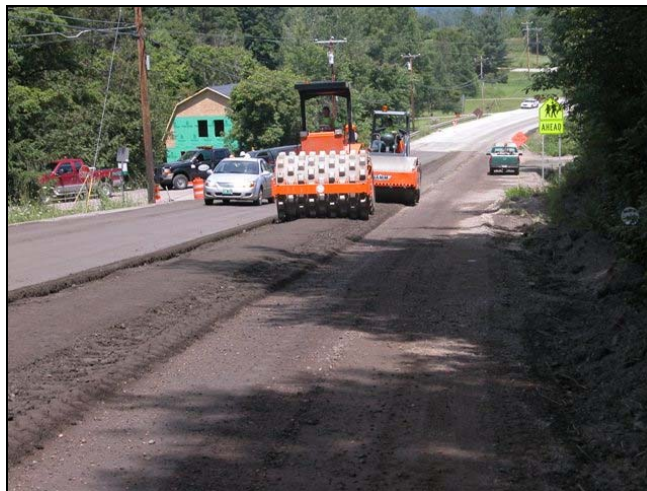
Figure 5 – Reclaimed Base Compaction
