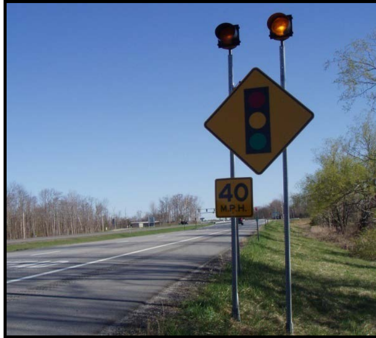
Figure 11 Typical Advanced Warning Flasher (AWF)
