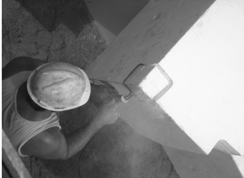
**Figure 3.8 Trimming a GeoFoam Block.**
