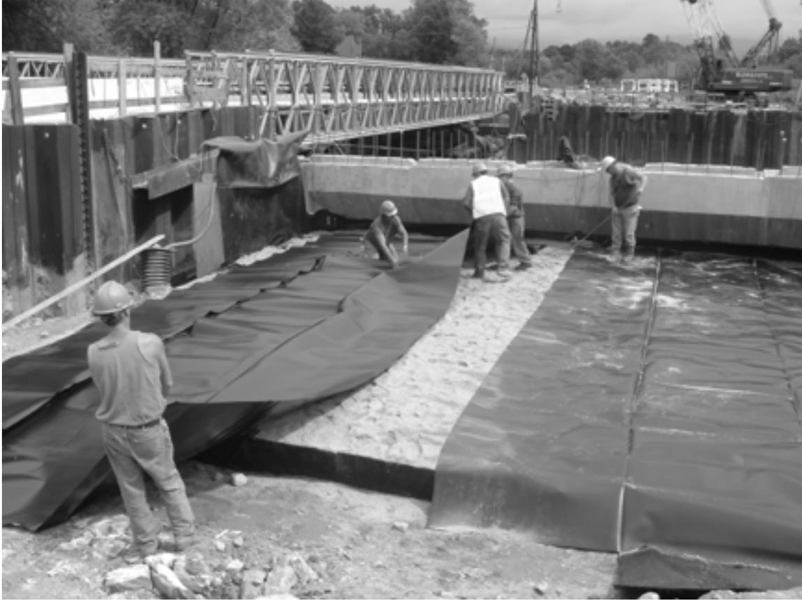
**Figure 3.13 Installation of Flexible PVC Geomembrane.**
