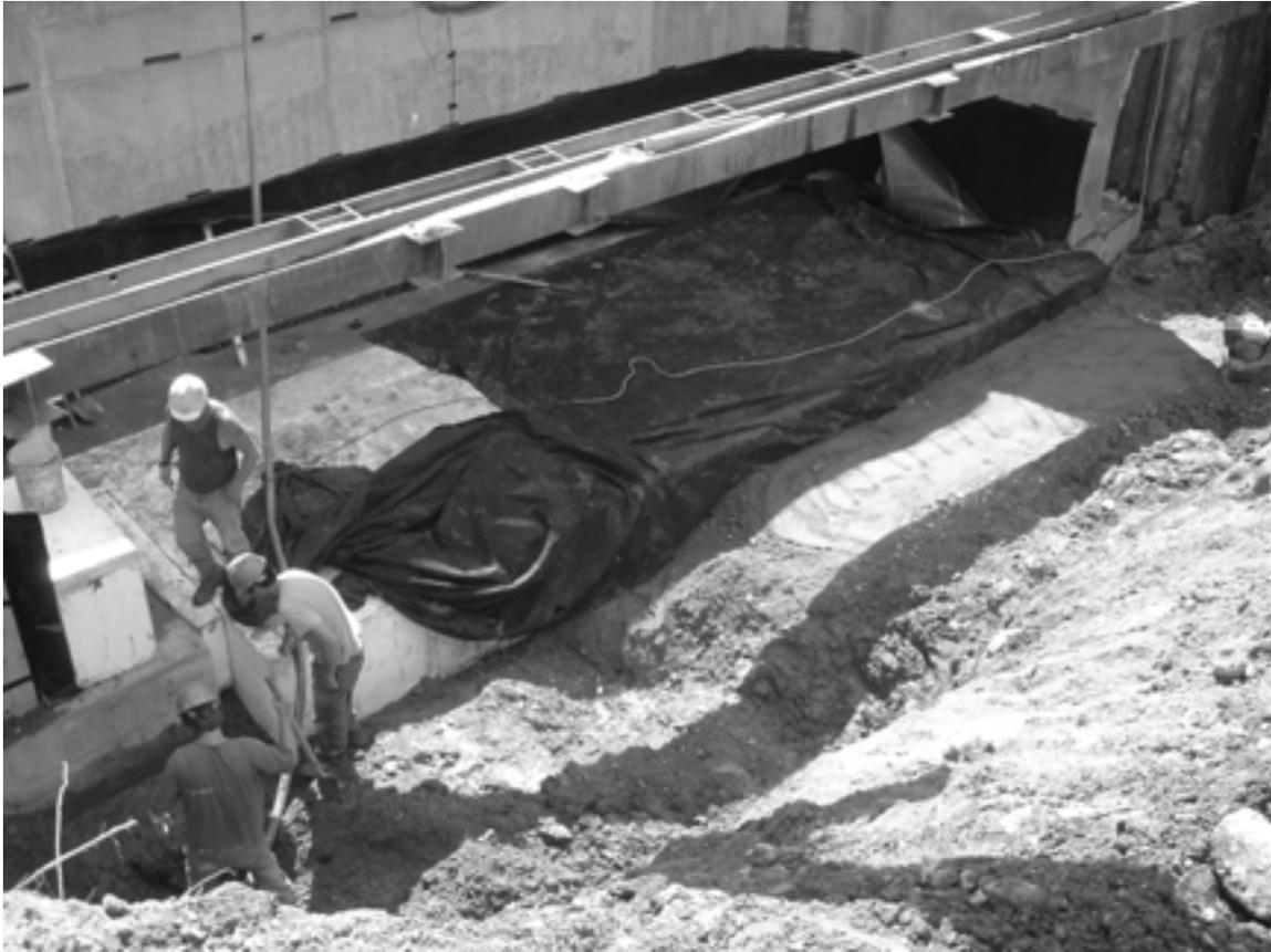
**Figure 3.10 Wrapping GeoFoam Blocks with Geotextile Separator and Backfilling.**
