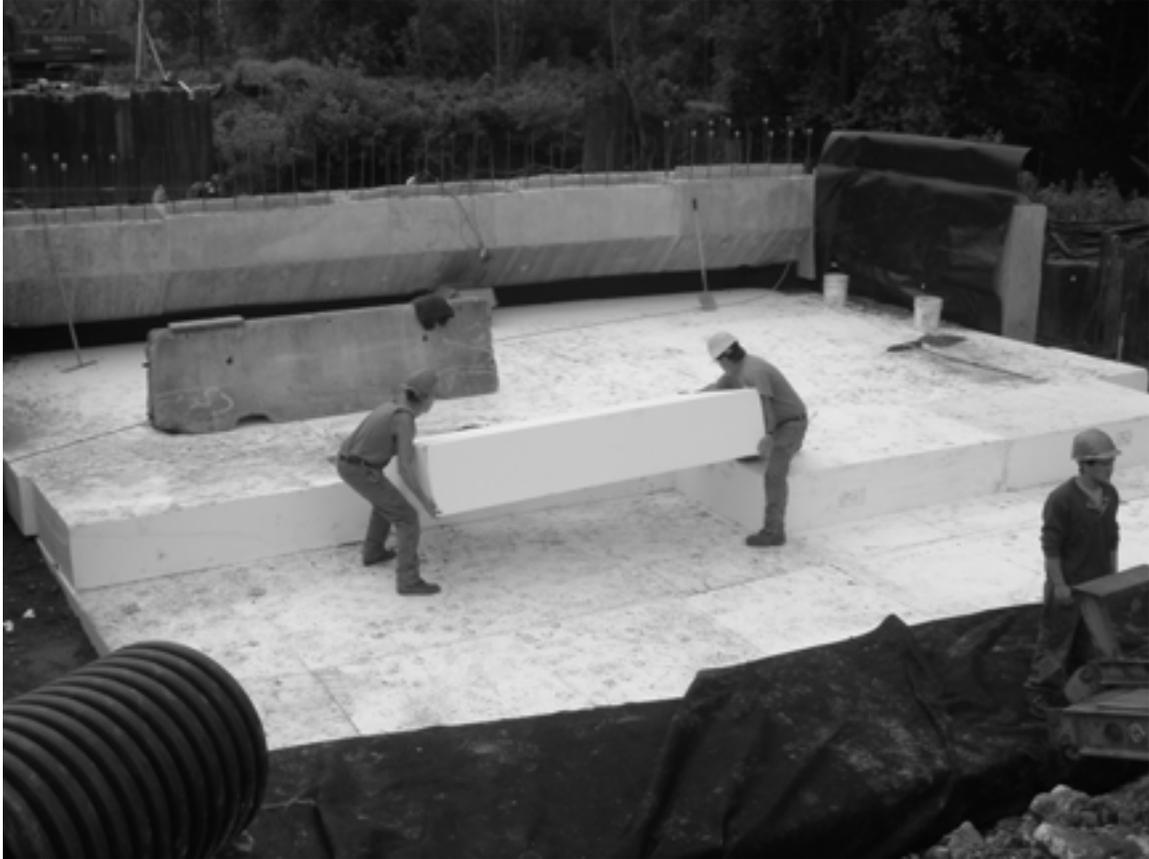
**Figure 3.11 Placement of GeoFoam Blocks in Stepped Layers.**
