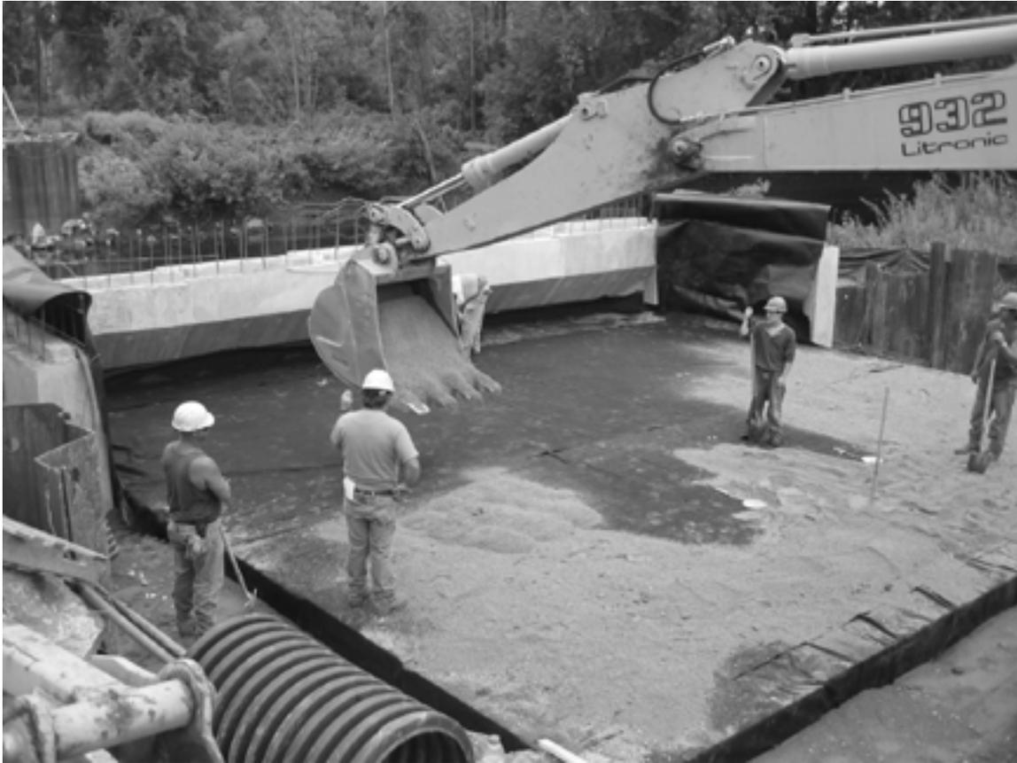
**Figure 3.12 Placement of Geotextile Separator and Tapered Sand Layer.**
