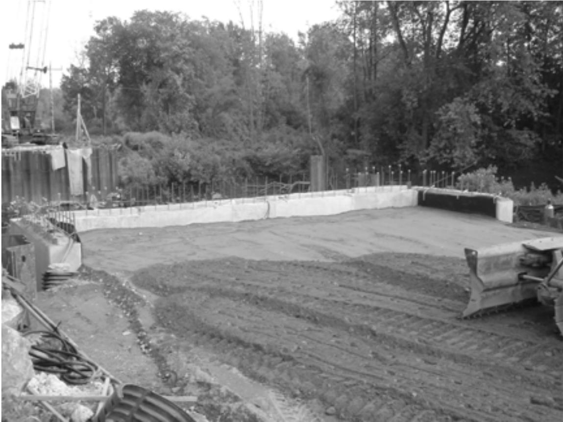
**Figure 3.14 Placement of Granular Backfill.**
